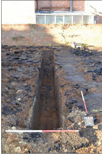
Plate 3. Trench foundation, looking north east, Scales: 2 x 1m.
