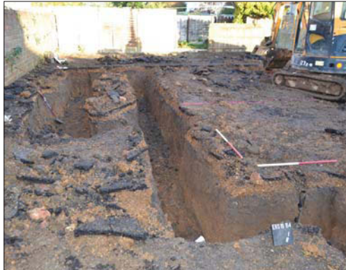
Plate 5. Trench foundation, looking south Scales: 2 x 1m.
