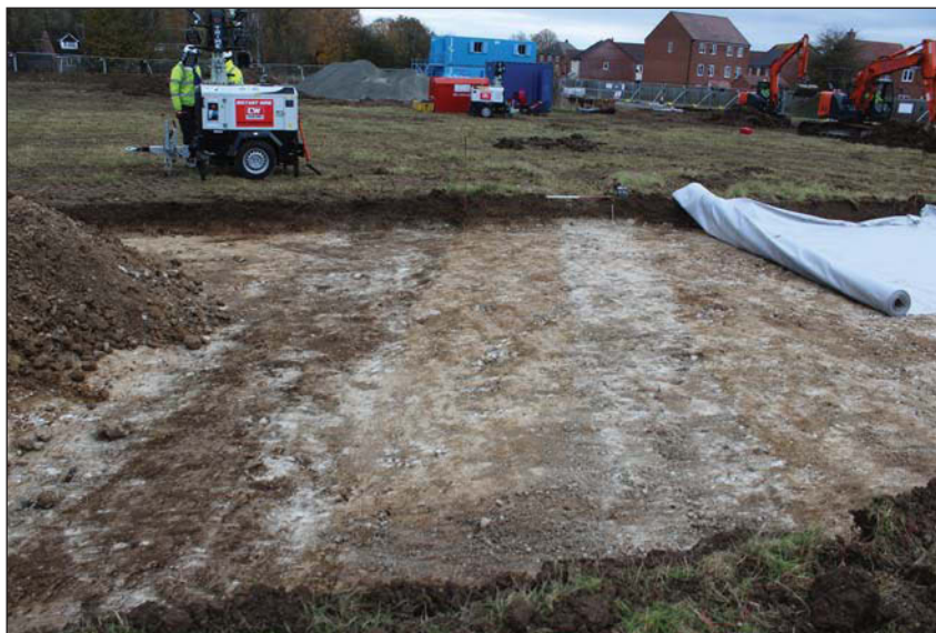
Plate 2. Access road, land drains, looking North East, Scales: 1m and 0.3m.
