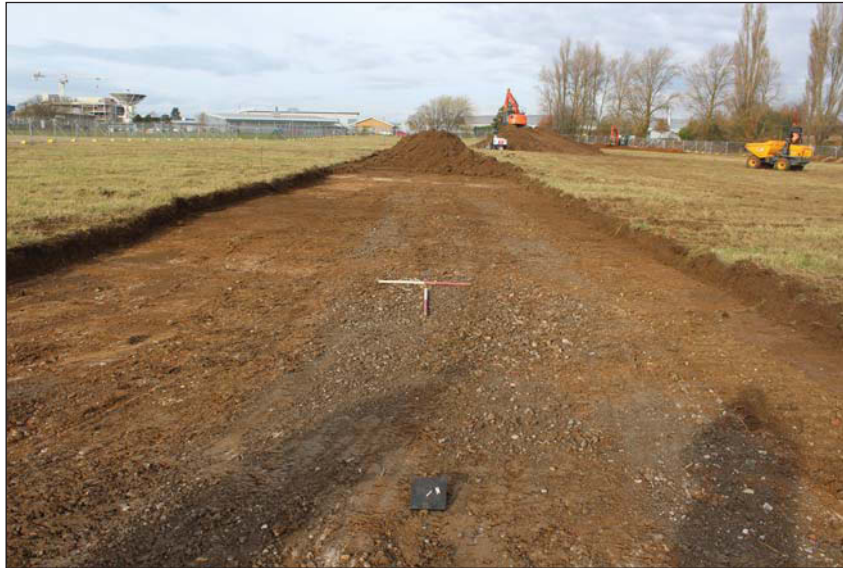
Plate 1. Temporary road access, looking North West, Scales: 2m and 1m.
