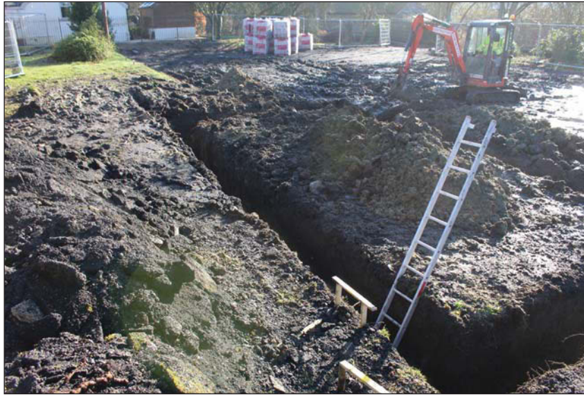
Plate 1. North area of new house footings, looking SE.
