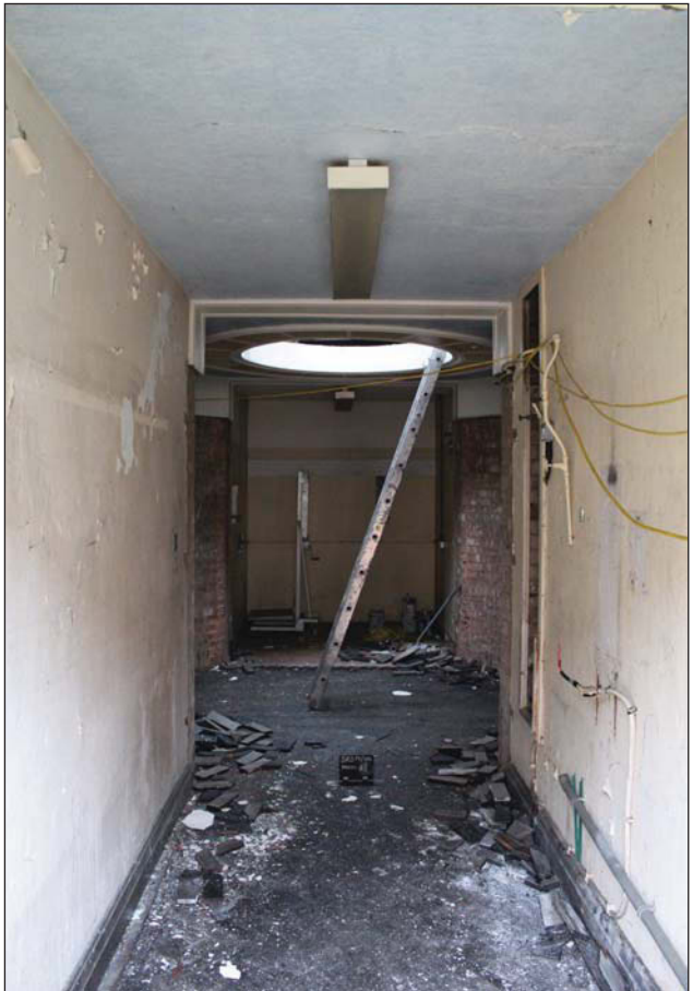
Plate 8. Internal corridor of 49, showing skylight, looking West
