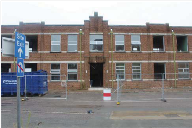
Plate 13. View of S end of 46, looking North-West
