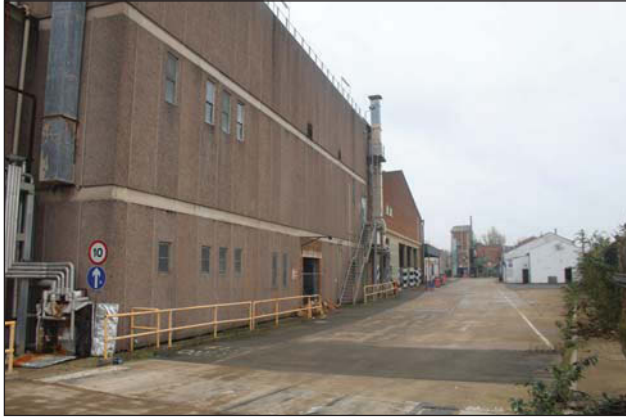
Plate 33. Exterior of 209, 20 and 29, looking North
