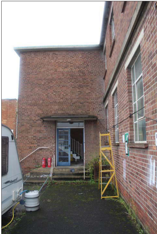
Plate 15. Building 111, looking East
