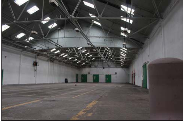
Plate 10. Interior of 145, looking East
