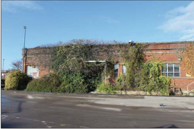
Plate 17. Building 107, east elevation, looking West
