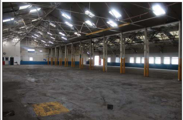
Plate 16. View of interior of 15, looking North-East
