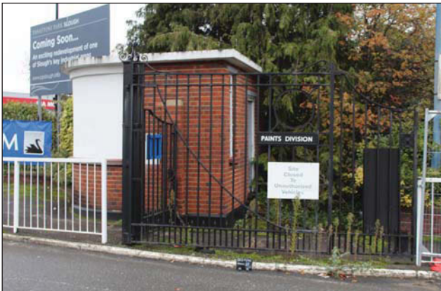
Plate 3. View of 115 and gate, looking north west.
