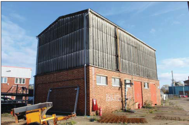
Plate 23. Building 188 looking North-West
