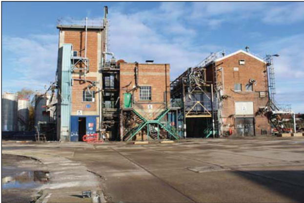
Plate 27. Buildings 190, 163, 201, south elevations, looking North.
