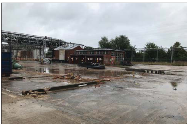
Plate 32. Buildings 60 and 150, looking North.
