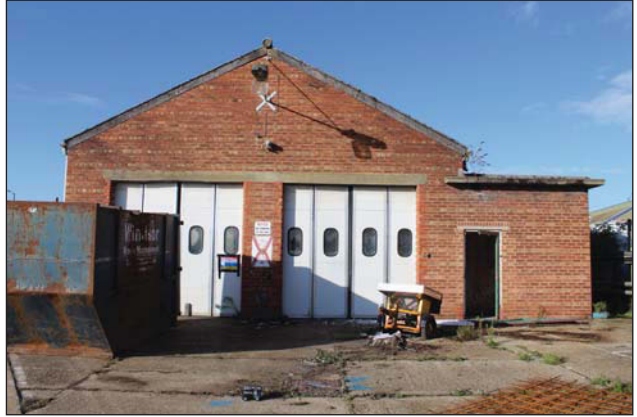
Plate 22. Building 173, looking West
