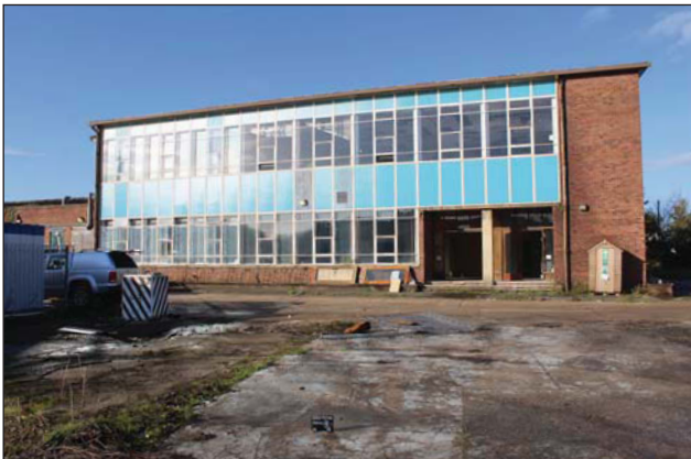
Plate 19. Building 107, northern addition, looking West
