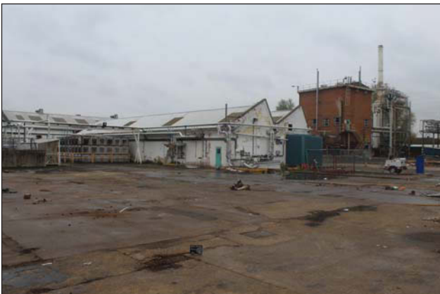
Plate 35. Building 24, looking North West
