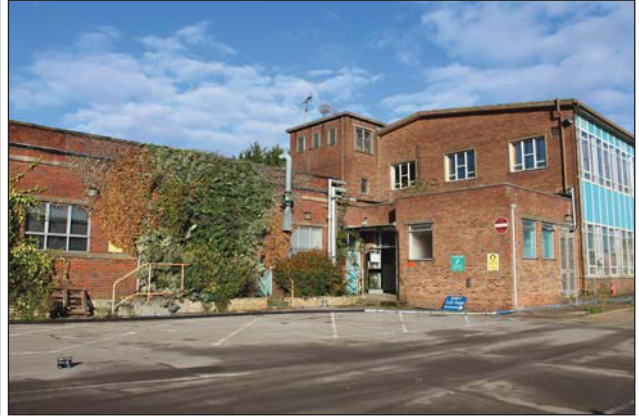
Plate 18. Building 107, east elevation showing northern addition, looking North-West
