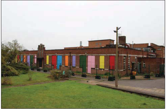
Plate 6. Oblique view of E and S ends of 49, looking East-North-East
