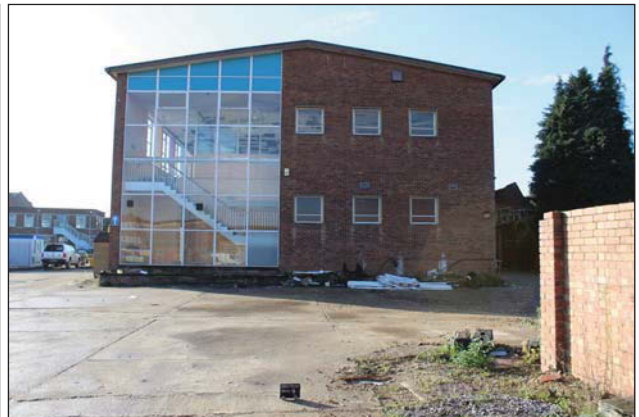
Plate 20. Building 107, northern elevation, looking South
