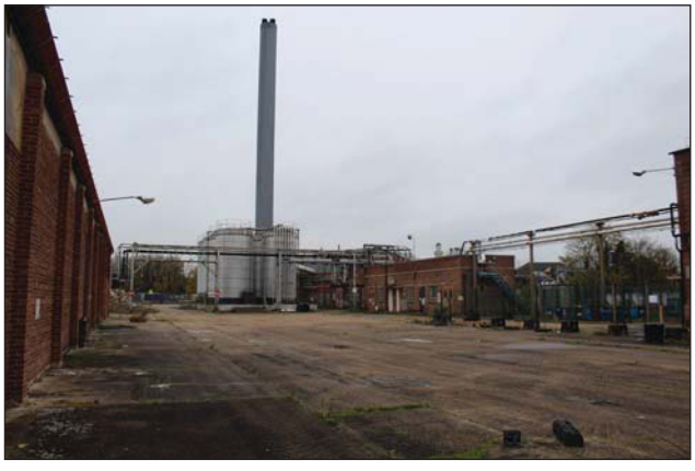
Plate 12. View alongside the S end of 145 towards storage tanks (217), looking East
