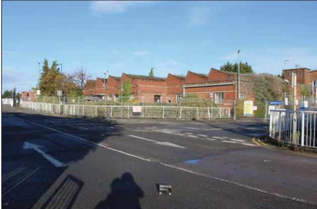
Plate 1. General view of site entrance and buildings 107 and 115, looking west
