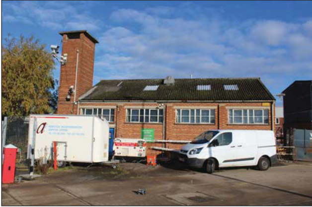
Plate 21. Building 173, looking North
