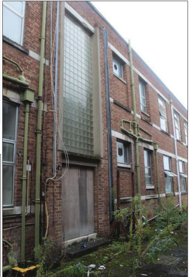
Plate 14. View of window detail of 46, looking South-West
