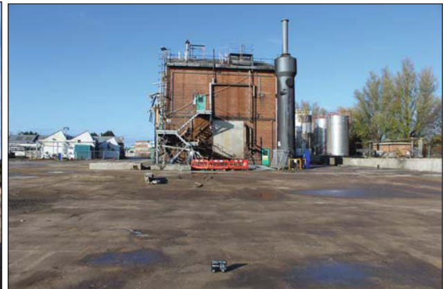
Plate 28. Building 201, east elevation, looking West.
