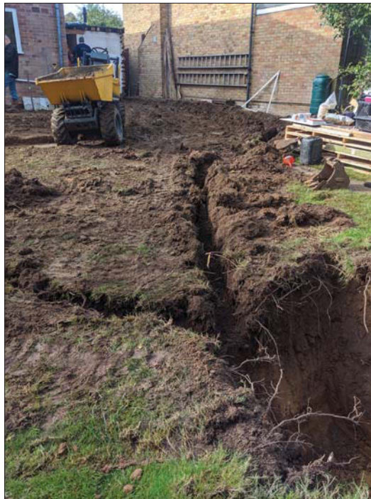
Plate 4. General view of site, looking North West
