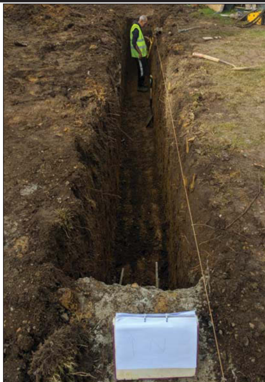
Plate 1. Footing, looking North
