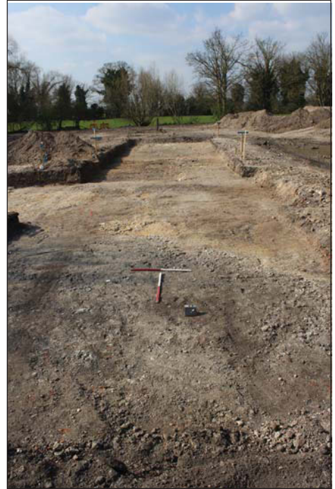
Plate 2. Working shot - deposit (58) in foreground, looking North West, Scales: 2x1m
