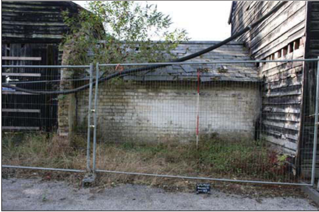
Plate 81. South elevation , looking S, Scales: 1x1m, 1x2m.
