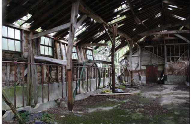
Plate 70. Interior along building, looking SE.
