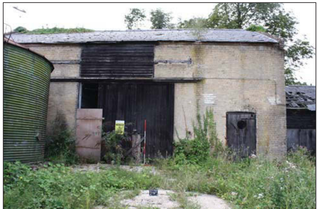
Plate 40. East elevation, looking W, Scales: 1x1m, 1x2m.
