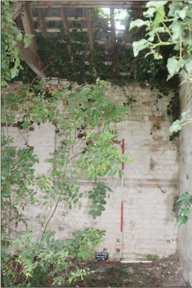
Plate 37. Rear wall, looking W, Scales: 1x1m, 1x2m.
