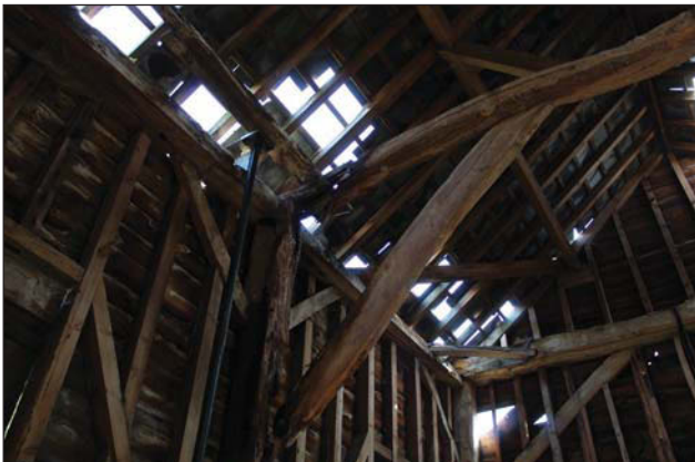
Plate 11. Brace detail on truss between bays 3 and 4, looking NE.
