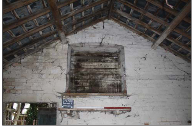
Plate 58. Internal window in wall, looking NW, Scales: 1x1m.
