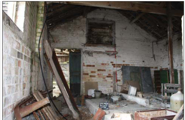
Plate 56. Along interior of building, looking NW, Scales: 1x1m, 1x2m.
