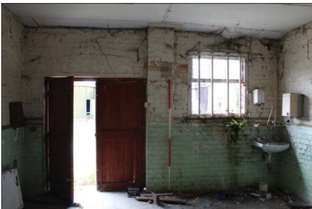
Plate 31. Room 5, door and window detail, looking S, Scales: 1x1m, 1x2m.
