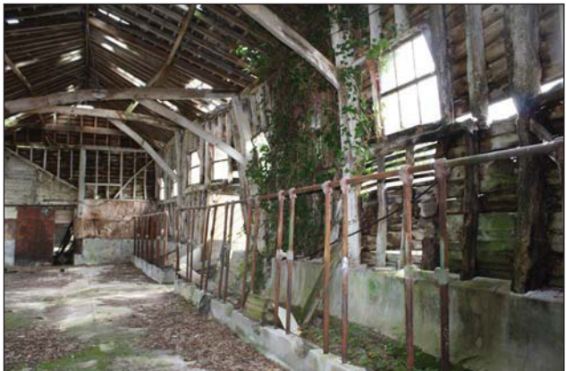
Plate 68. Interior along building, looking SW.
