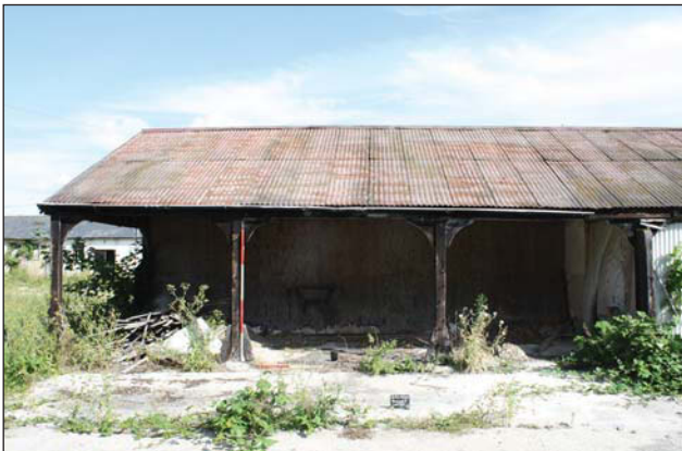
Plate 87. South elevation, west end, looking N, Scales: 1x1m, 1x2m.
