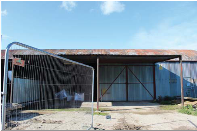
Plate 89. North end, Eastern elevation of building, looking W, Scales: 1x1m.
