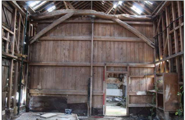
Plate 18. Partition between bays 2 and 3, looking E, Scales: 1x1m, 1x2m.
