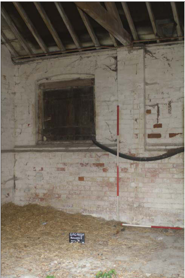
Plate 27. Room 2, rear wall, west end, looking N, Scales: 1x1m, 1x2m.
