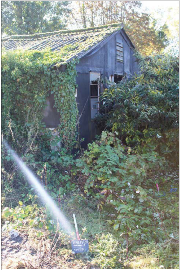
Plate 96. General corner view of North of building, looking S, Scales: 1x1m.
