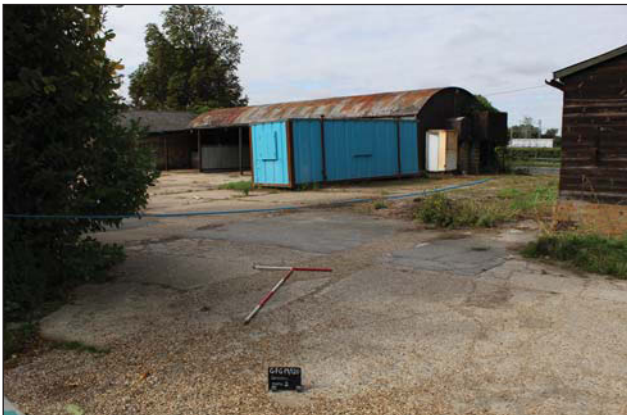
Plate 3. View to barn B, looking SW, Scales: 1x1m, 1x2m
