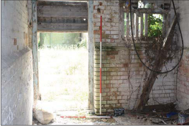
Plate 29. Room 4, door and window detail, looking S, Scales: 1x1m, 1x2m.
