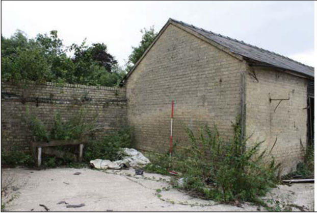
Plate 49. East gable end, looking SW, Scales: 1x1m, 1x2m.
