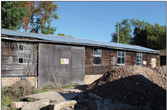
Plate 92. General view of South side of building, looking N, Scales: 1x1m.
