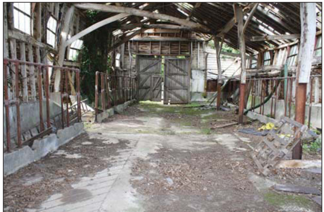
Plate 76. Interior view along building, showing flooring, looking N.
