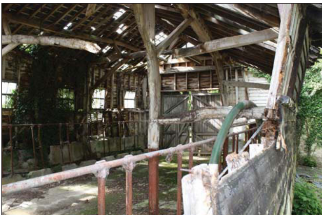
Plate 71. Interior elevation North end of barn looking N.
