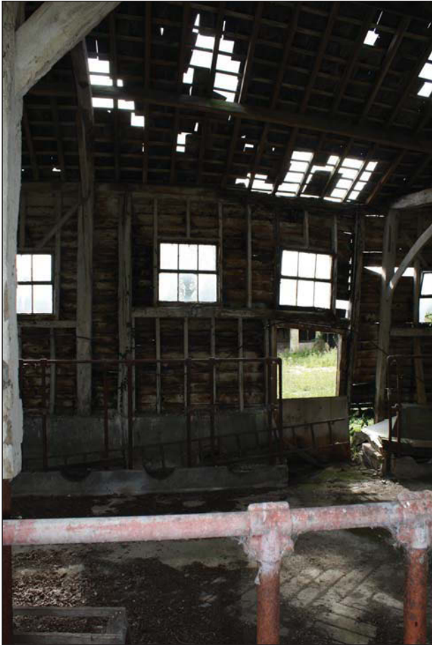
Plate 69. Interior west elevation, centre, looking W.
