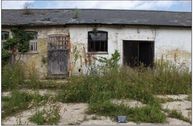
Plate 22. South elevation, centre, looking N, Scales: 1x1m, 1x2m.
