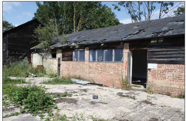
Plate 52. Along building, looking NE, Scales: 1x1m, 1x2m.
