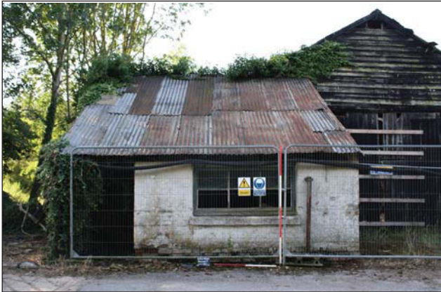
Plate 77. North elevation, looking S, Scales: 1x1m, 1x2m.
