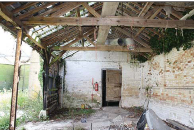
Plate 39. Internal wall between buildings 4 and 5, looking S, Scales: 1x1m, 1x2m.
