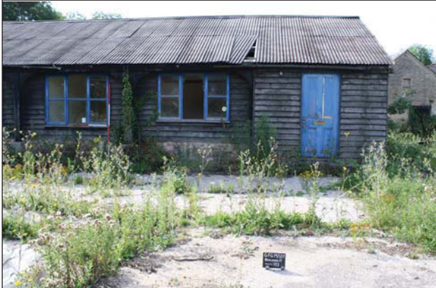
Plate 85. North elevation, West end, looking S, Scales: 1x1m, 1x2m.
