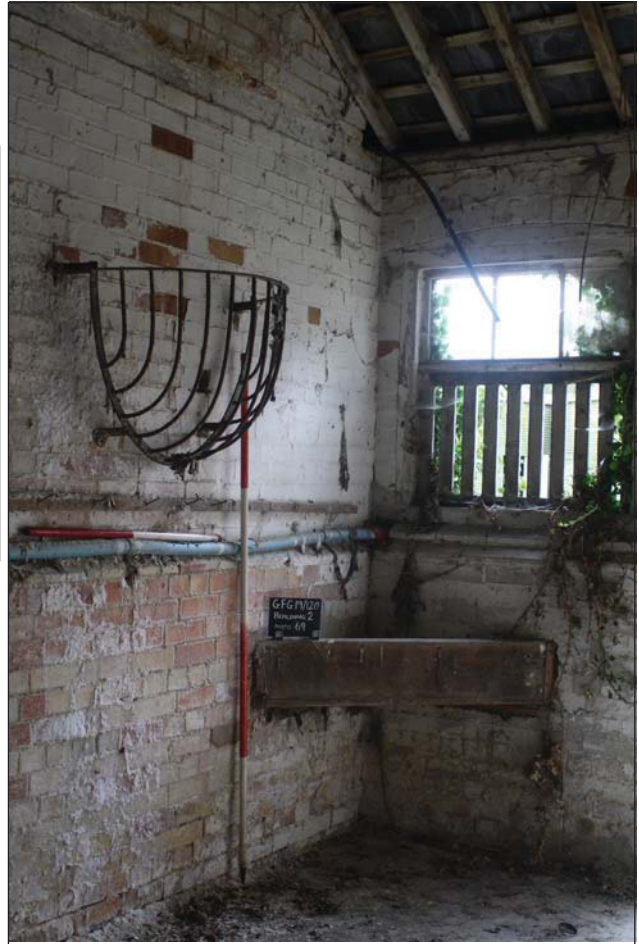
Plate 30. Room 3, window, trough and hay basket, looking SE, Scales: 1x1m, 1x2m.
