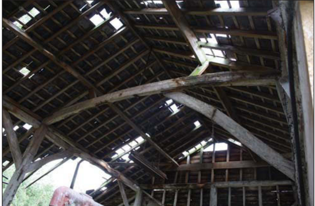
Plate 66. Interior, roof apex, South end, looking S.
