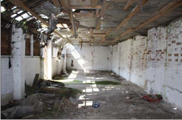
Plate 53. Along interior of building, looking NW, Scales: 1x1m, 1x2m.
