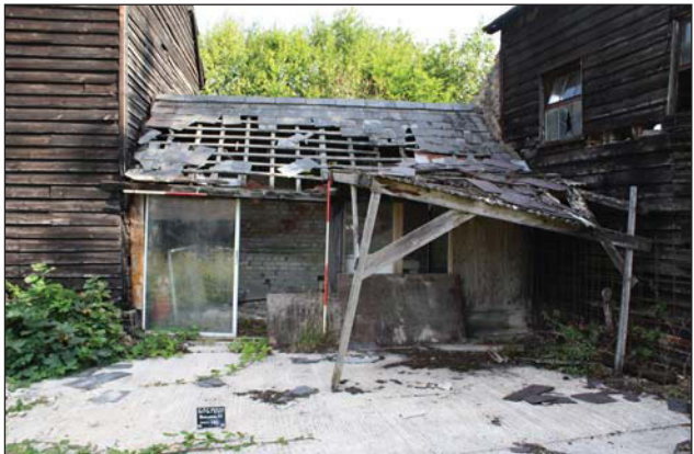
Plate 80. North elevation, looking N, Scales: 1x1m, 1x2m.
