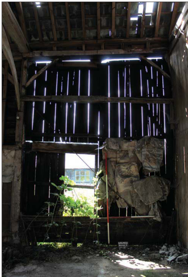
Plate 17. Bay 3 door detail, looking S, Scales: 1x1m, 1x2m.
