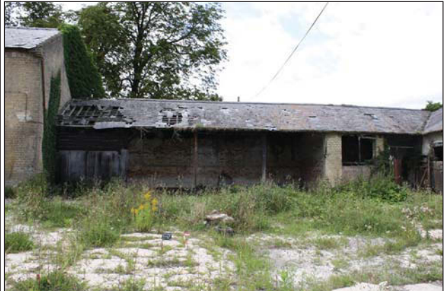
Plate 38. General view of building, looking W, Scales: 1x1m, 1x2m.
