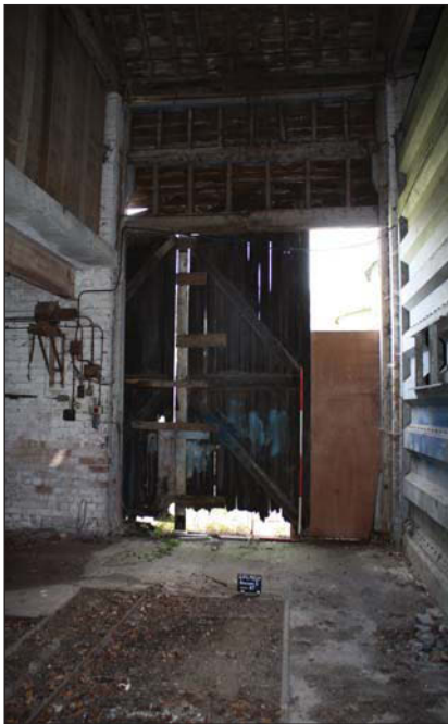
Plate 43. Door detail, looking E, Scales: 1x1m, 1x2m.
