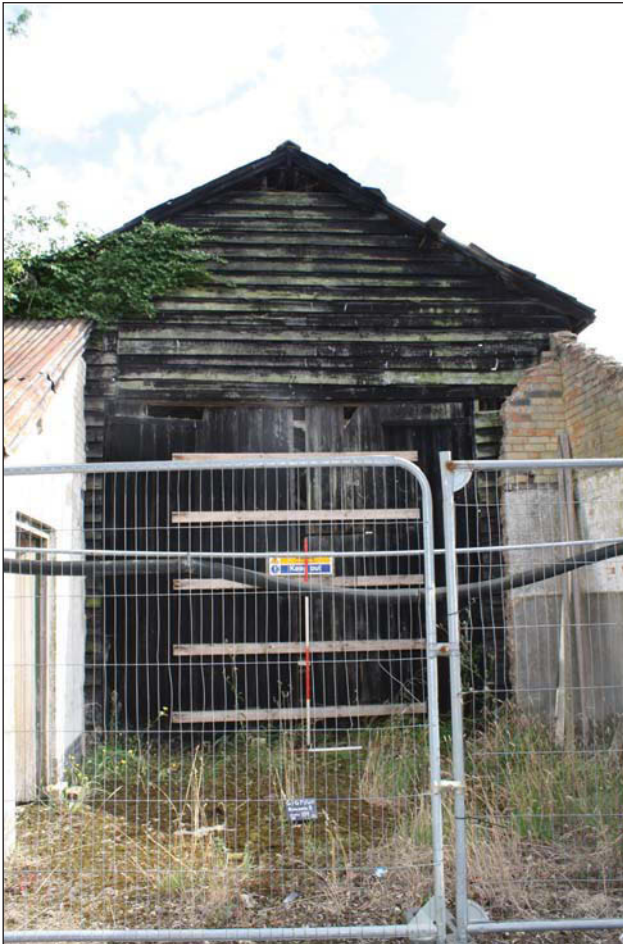
Plate 61. Elevation of North end of building, looking S, Scales: 1x1m, 1x2m.
