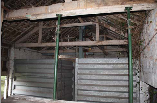
Plate 45. Truss detail, looking S.
