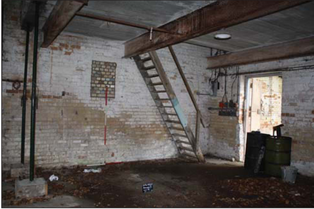
Plate 41. View to stairs, looking NW, Scales: 1x1m, 1x2m.
