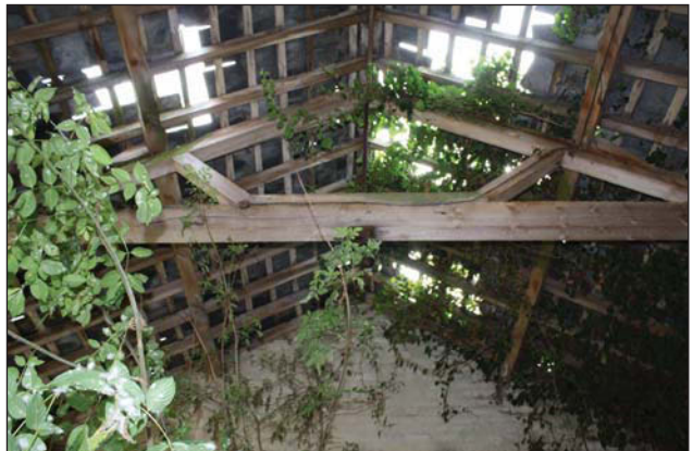
Plate 36. Truss detail, looking S.
