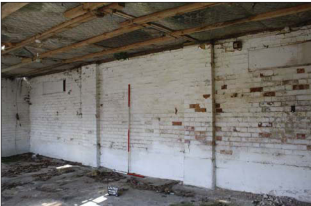
Plate 55. Wall detail, looking NE, Scales: 1x1m, 1x2m.
