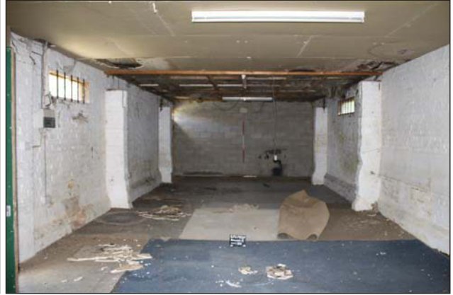
Plate 50. Modern partition wall, looking SW, Scales: 1x1m, 1x2m.
