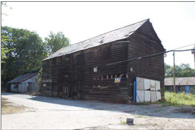
Plate 7. Oblique view north and west elevations, looking SE, Scales: 1x1m, 1x2m.
