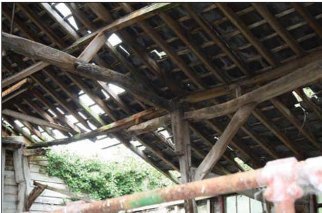
Plate 67. Replaced roof supports, looking NE.
