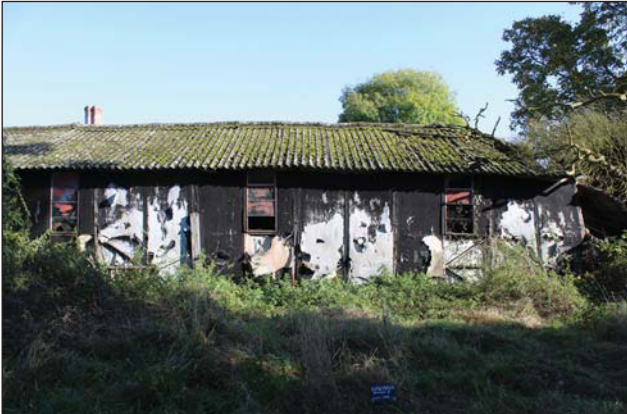
Plate 95. General view of SW of building, looking NE, Scales: 1x1m.
