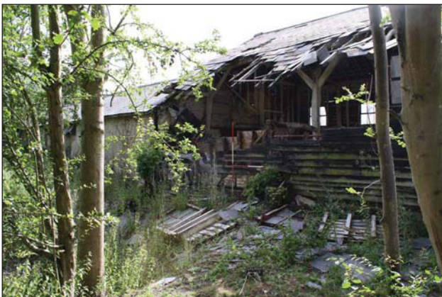
Plate 63. West elevation, South end, looking S, Scales: 1x1m, 1x2m.
