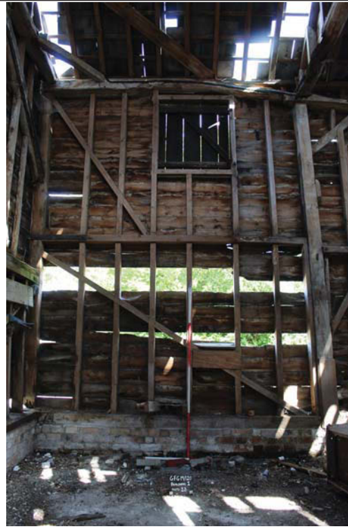
Plate 6. Bay 1 timber framing detail, looking N, Scales: 1x1m, 1x2m.
