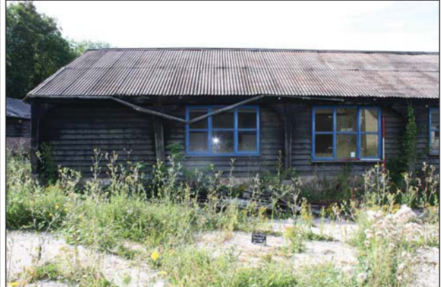
Plate 86. North elevation, East end, looking S, Scales: 1x1m, 1x2m.
