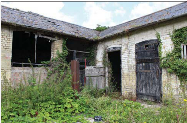
Plate 35. Oblique view of buildings 2 and 3, looking NW, Scales: 1x1m, 1x2m.
