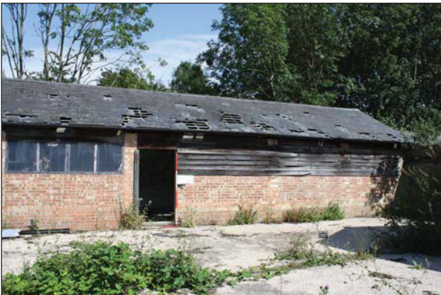
Plate 51. West elevation, looking SE, Scales: 1x1m, 1x2m.
