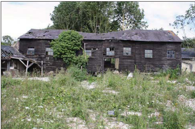
Plate 59. General view, looking NE, Scales: 1x2m.
