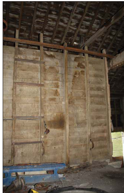
Plate 44. Partition detail, looking E.
