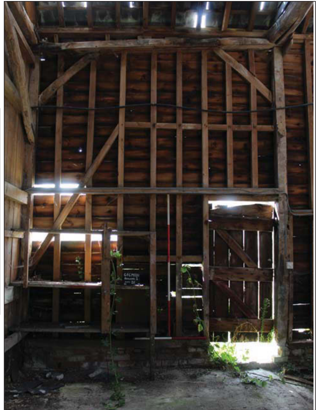
Plate 10. Bay 2 timber framing detail, looking S, Scales: 1x1m, 1x2m.
