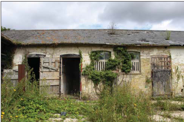
Plate 23. South elevation, west end, looking N, Scales: 1x1m, 1x2m.
