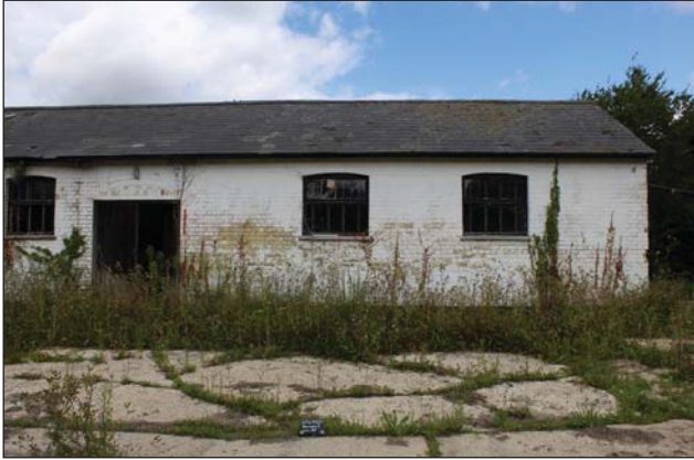
Plate 21. South elevation, east end, looking N, Scales: 1x1m, 1x2m.
