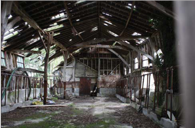
Plate 65. Interior along building, South elevation, looking S.
