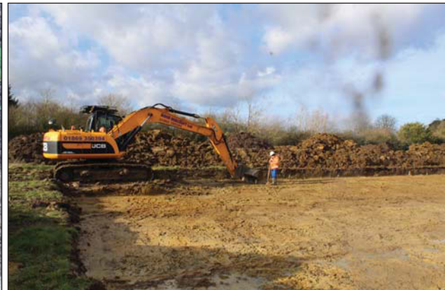
Plate 4. Working shot, looking West.
