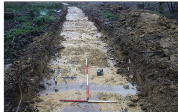
Plate 10. Trench 40, looking North. Scales: 2m, 1m and 0.50m.
