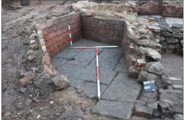
Plate 26. Storage room (fill 67) and Stone floor (81), looking north-east, Scales: 2m, 1m and 1m.
