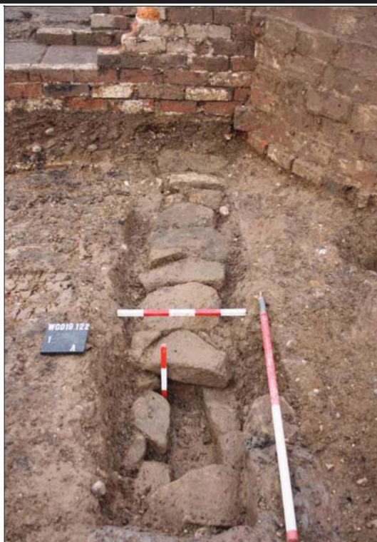
Plate 19. Stone-lined drainage channel [1] before full excavation, looking north, Scales: 1m, 0.5m and 0.3m.
