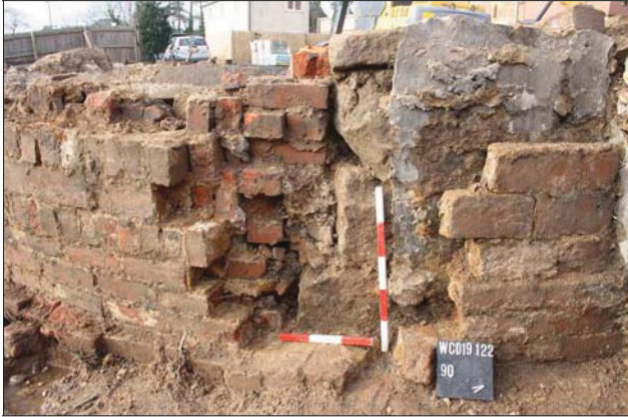
Plate 11. Repair to windmill (90), looking north-west, Scales: 0.5m and 0.3m.
