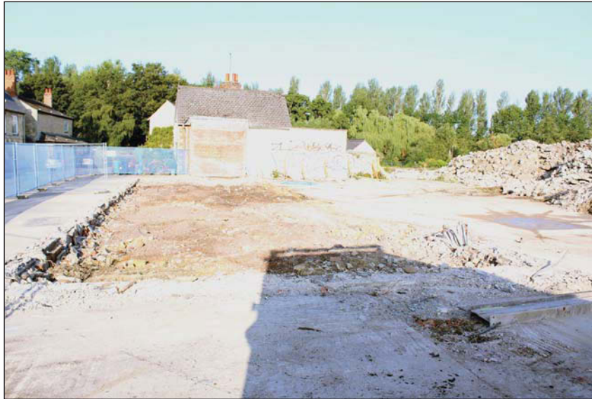
Plate 9. Location of office block after demolition to foundation, looking west.
