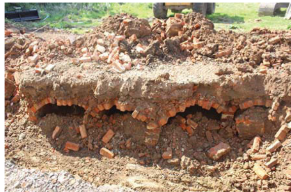
Plate 10. Segment of vaults, looking north-north-east, situated at the western end of the proposed academy building's footprint.
