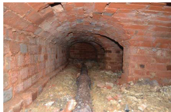
Plate 12. Interior of vault with in-situ pipework, looking north
