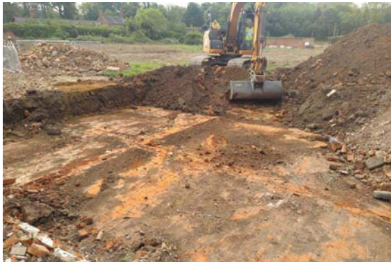
Plate 7. Area strip within former walled garden, looking SE
