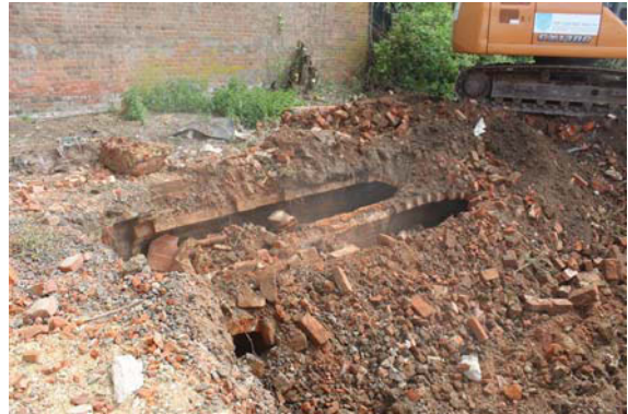
Plate 8. Vaults during exposure, NE corner of the Academy building footprint, looking South
