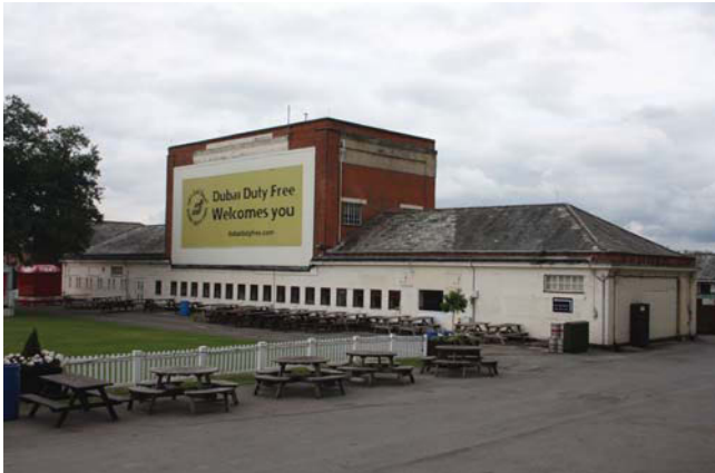
Plate 3. Oblique view of building, looking north-east, Scales: 2m and 1m.
