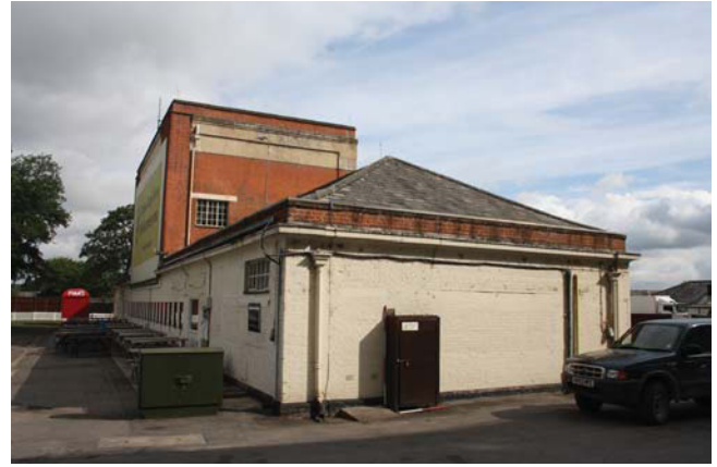
Plate 2. Oblique view of south wall, looking north-east, Scales: 2m and 1m.
