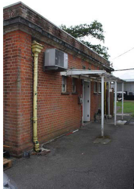
Plate 4. Oblique view, north end of building, looking south-west, Scales: 2m and 1m.
