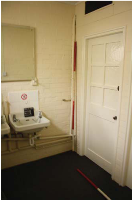
Plate 13. Room 16: toilet door and sink (Ladies), looking north-west, Scales: 2m and 1m.
