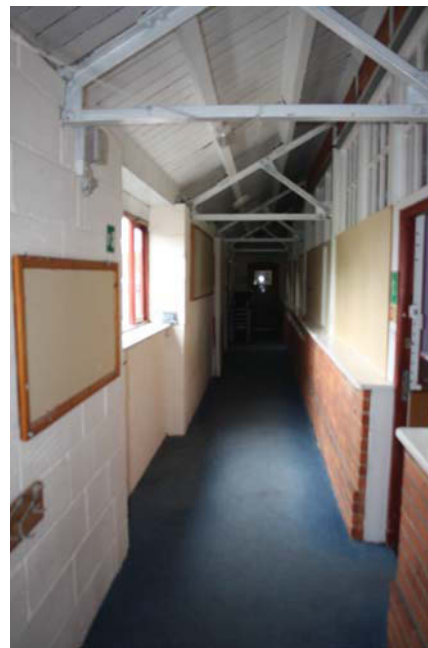
Plate 32. Nursery Room 14: view along corridor, looking south, Scales: 2m and 1m.
