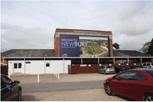
Plate 1. Overview of building, looking west Scales: 2m and 1m.
