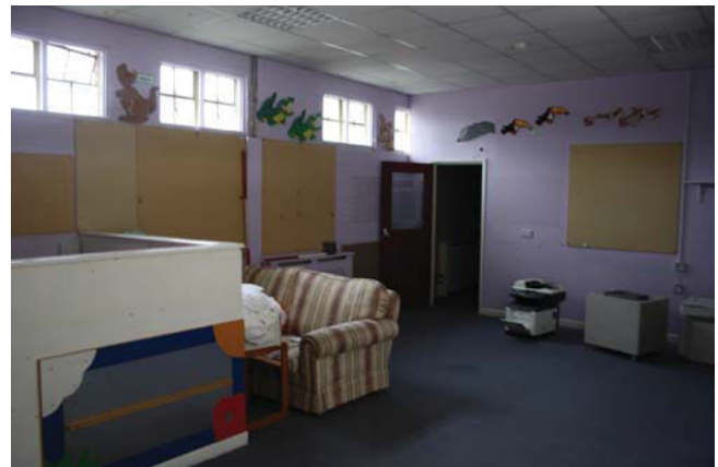
Plate 28. Nursery Room 2: general view to windows, looking north-east, Scales: 2m and 1m.
