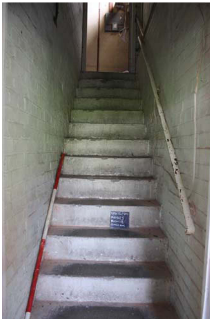
Plate 15. Room 18: stairs, looking east, Scale: 2m.
