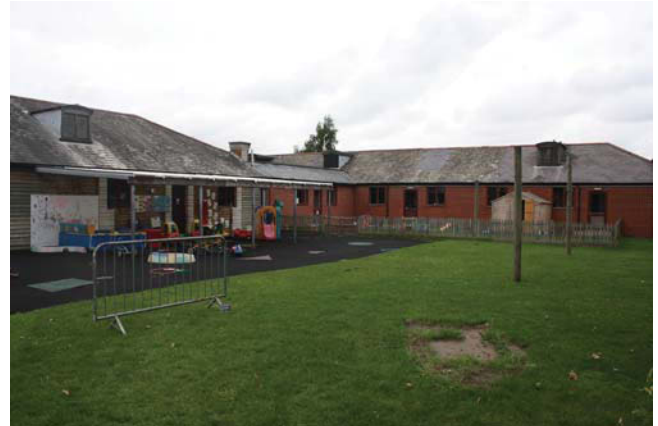
Plate 22. Nursery: east and south elevation, oblique, looking north-west, Scales: 2m and 1m.
