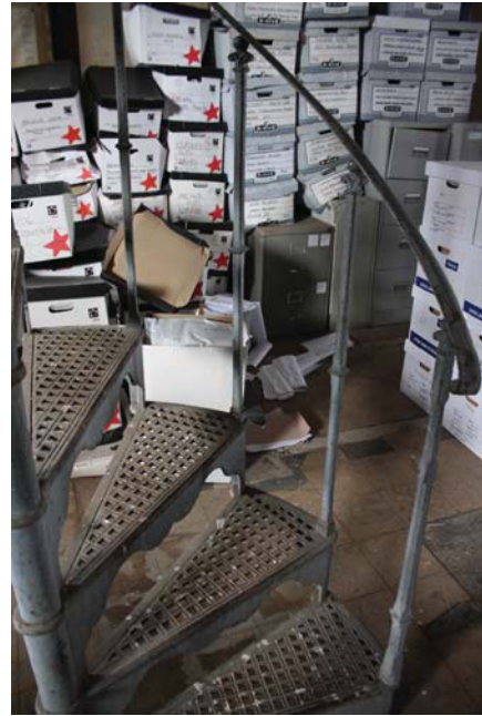
Plate 18. Room 18: detail of spiral staircase, looking west.
