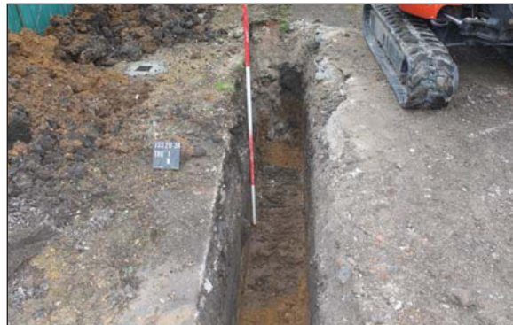
Plate 9. Trench 6, looking South. Scale: 2m.
