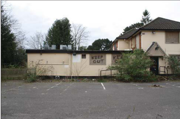
Plate 5. Northeast facing elevation, looking southwest, Scales: 2 x 1m.
