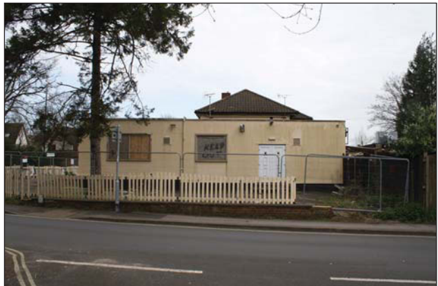
Plate 8. Southwest facing elevation, looking northeast.
