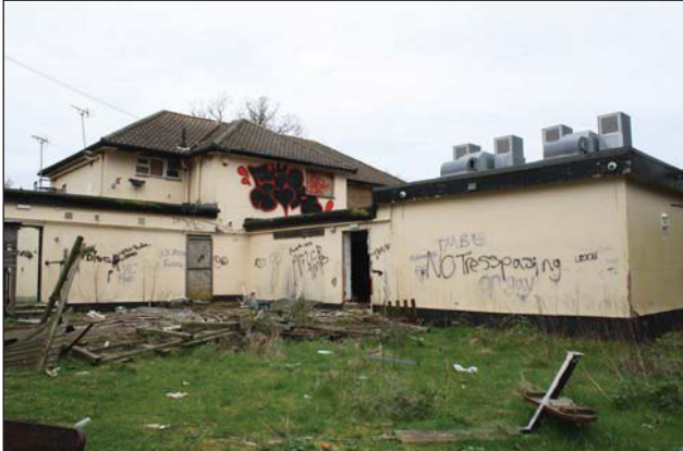
Plate 9. Oblique of rear of building, looking northeast, Scales: 2 x 1m.
