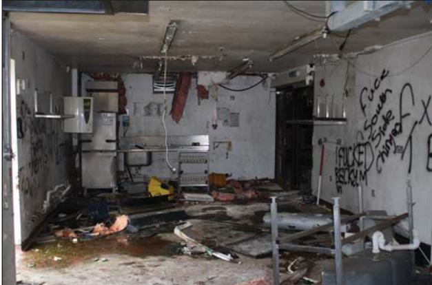
Plate 21. Room 12, kitchen, looking north, Scales: 2 x 1m.
