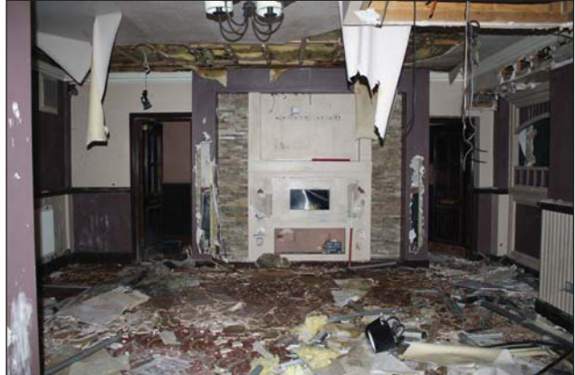
Plate 18. Room 7, view to toilets, looking northeast, Scales: 2 x 1m.
