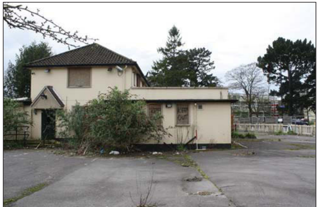
Plate 4. Northeast facing elevation, looking southwest, Scales: 2 x 1m.
