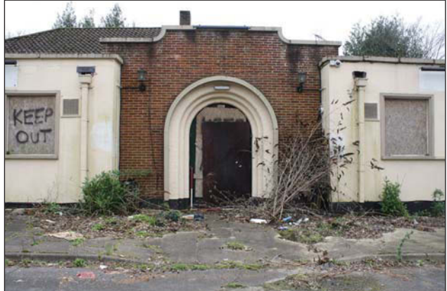
Plate 2. Main entrance detail, looking southeast, Scales: 2 x 1m.
