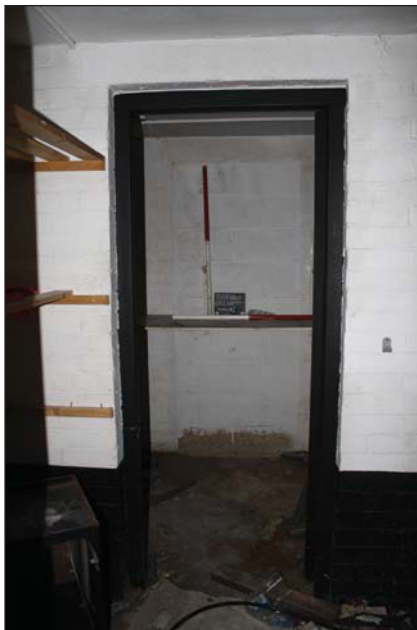
Plate 11. Room 2, blocked door, looking southeast, Scales: 2 x 1m.
