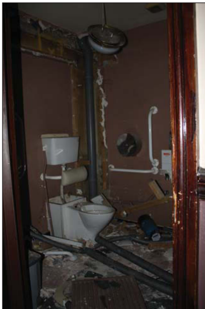
Plate 27. Room 14, disabled toilet, looking southeast.
