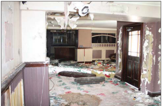
Plate 16. Room 11, family bar, looking northwest, Scales: 2 x 1m.
