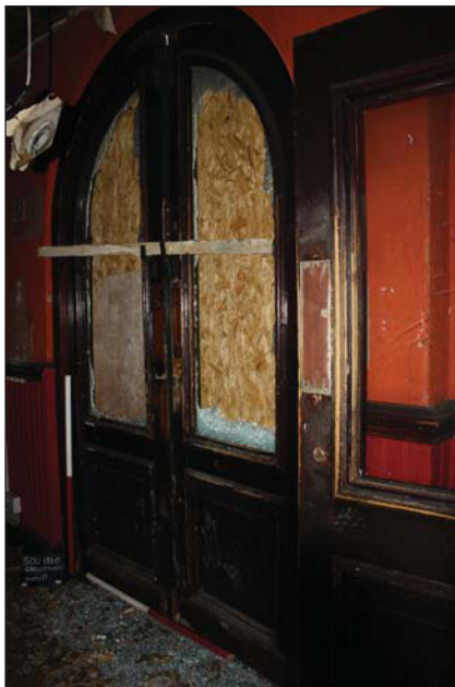
Plate 3. Main doors, looking west, Scales: 2 x 1m.
