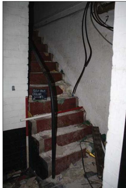
Plate 10. Room 1, view to stairs, looking southwest, Scales: 2 x 1m.
