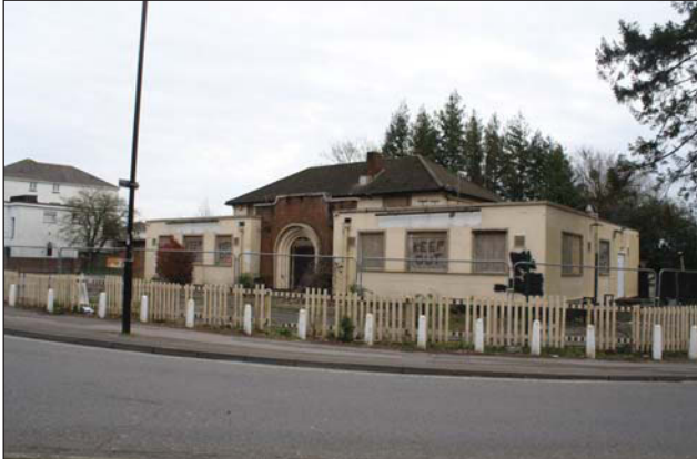
Plate 1. Oblique of frontage , looking southeast
