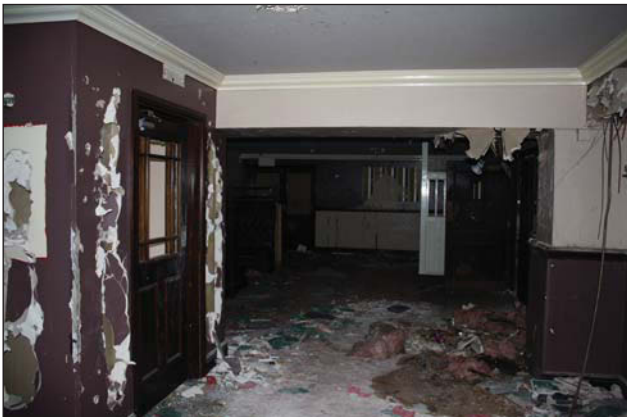
Plate 15. Room 7, family bar, looking southeast, Scales: 2 x 1m.
