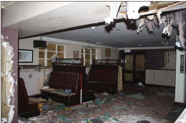
Plate 19. Room 11, family bar, looking southeast, Scales: 2 x 1m.
