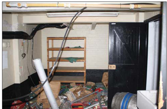
Plate 12. Room 3, looking northeast.
