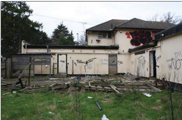
Plate 7. Rear of building, looking northwest, Scales: 2 x 1m.
