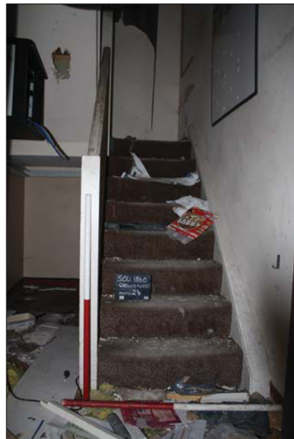
Plate 28. Room 15, stairs to first floor, looking northeast, Scales: 2 x 1m.
