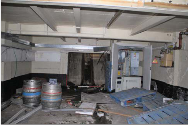
Plate 13. Room 5, view to barrel slide, looking southwest, Scales: 2 x 1m.
