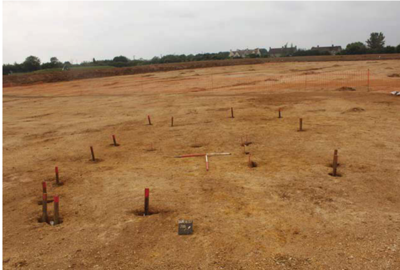
Plate 7: View of structure 1021 looking North West, Scales: 1m
