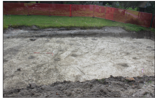
Plate 2. General view of southern part of excavation area, looking East.
