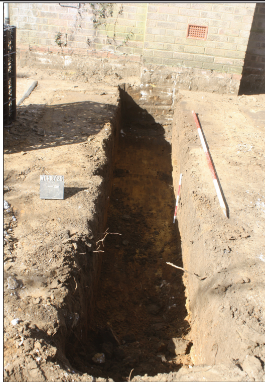
Plate 3. Foundation trench, looking west, Scales: 2m and 0.5m.
