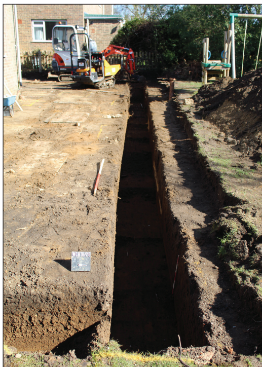
Plate 1. New southern footing, looking E, Scales: horizontal 1m, vertical 0.5m.
