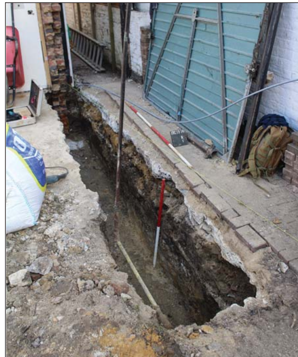
Plate 4. Eastern footing trench, looking North-east. Scales: 2m and 1m.
