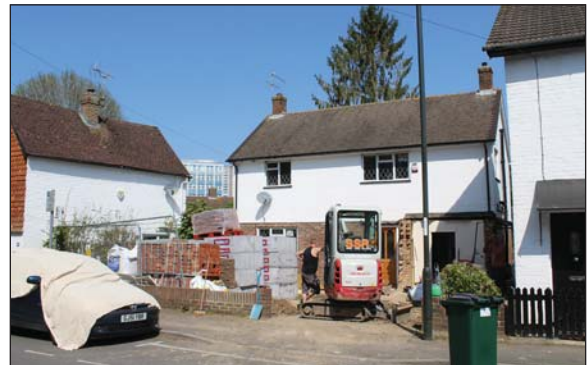
Plate 8. General view of site, looking North
