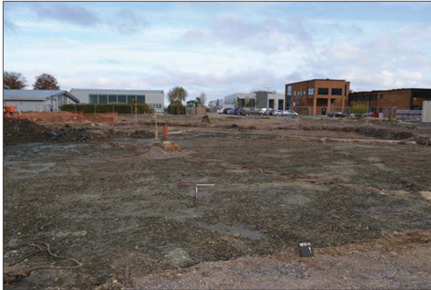
Plate 3. Car park, general shot over reduced area, looking north north east, Scales: 2m and 1m.
