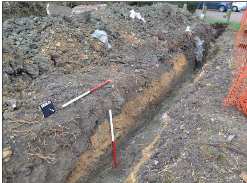
Plate 4. Service trench 1, looking south west, Scales: 1m.
