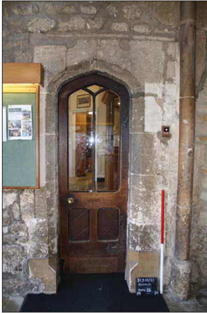
Plate 8. Door detail, looking Southeast, Scales: 1x1m.
