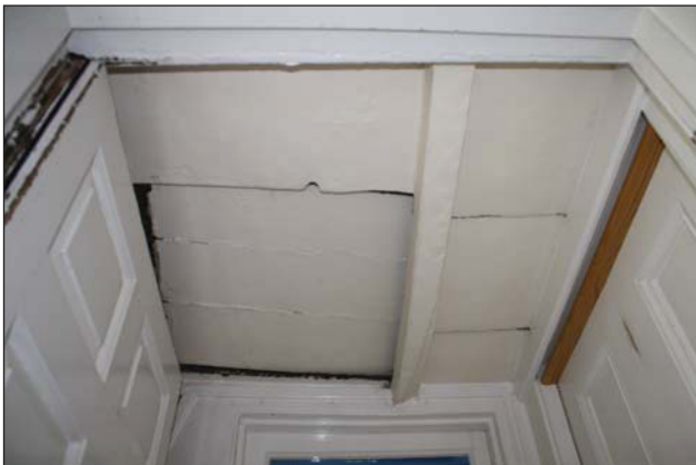
Plate 25. Room 2, ceiling detail looking Northeast.
