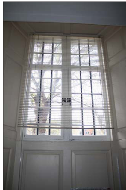
Plate 38. Room 4, window detail, looking Southwest.
