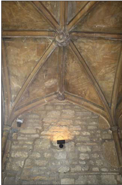
Plate 4. Top of arch detail, looking Southeast.
