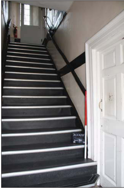
Plate 23. Room 2, oblique of stairs showing timber framing, looking West, Scales: 1m.
