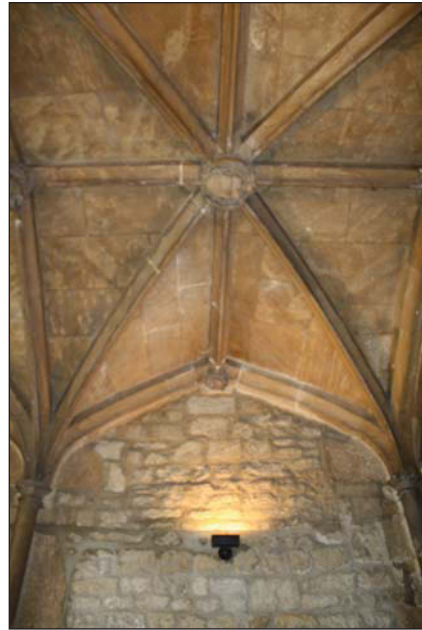
Plate 5. Top of arch detail, looking Southeast.
