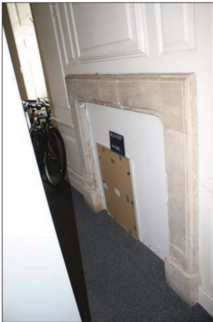
Plate 41. Room 4, fireplace detail, looking Southeast.
