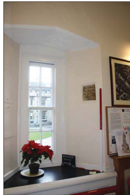
Plate 18. Room 1, window and plaque detail, looking East, Scales: 1m and 0.3m.
