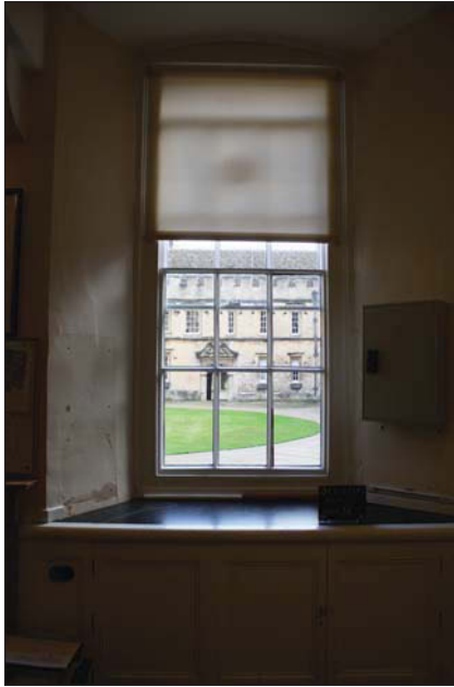
Plate 19. Room 1, window detail, looking Northeast, Scales: 1m and 0.3m.
