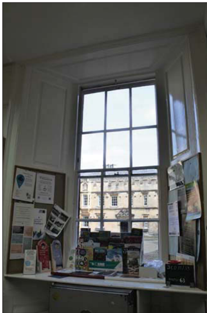
Plate 33. Room 3, window detail, looking Northeast, Scales: 1m.
