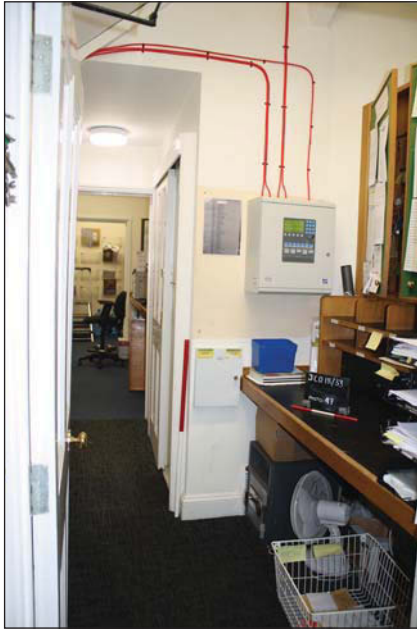
Plate 27. Room 2b, view along corridor, looking Southeast, Scales: 1m and 0.3m.
