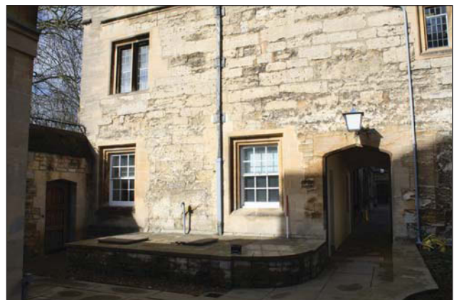
Plate 14. South elevation, oblique, looking West, Scales: 2x1m.
