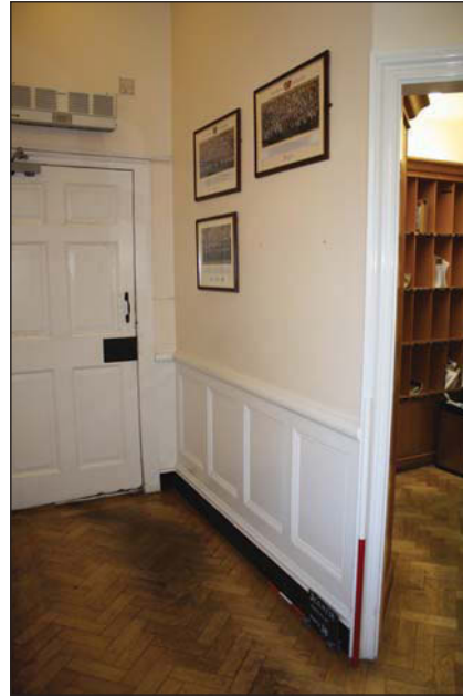
Plate 16. Room 1, oblique of panelling, looking South, Scales: 1m and 0.3m.
