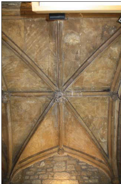
Plate 10. Vault roof detail, looking Northwest.
