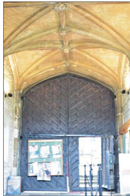
Plate 3. Archway, door and vaulted ceiling detail, looking Southwest, Scales: 2x1m.
