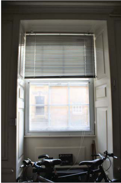
Plate 39. Room 4, window detail, looking Southeast.
