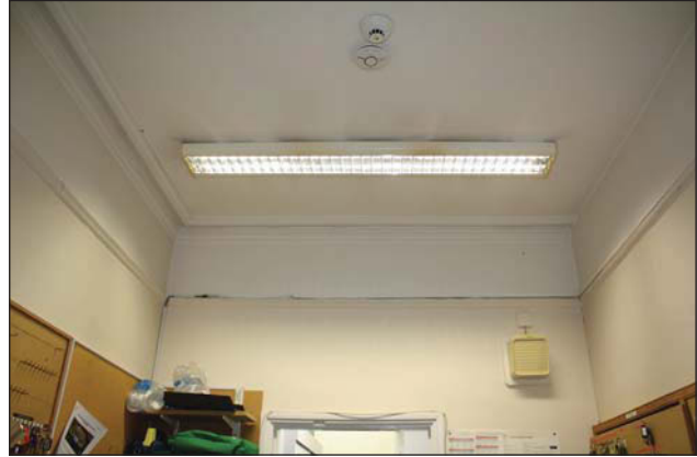
Plate 32. Room 3, coving detail, looking Northwest.
