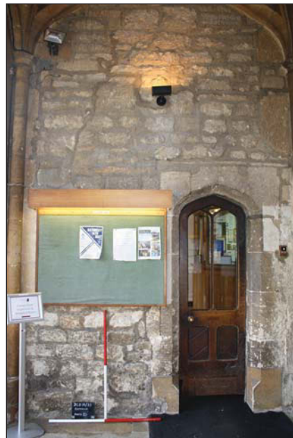
Plate 7. Door detail, looking Southeast, Scales: 2x1m.
