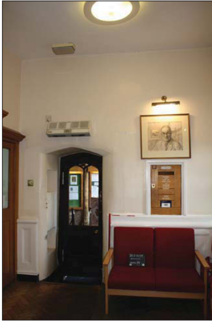
Plate 15. Room 1, North wall, looking Northwest, Scales: 1m and 0.3m.
