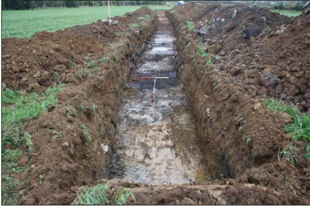
Plate 1. Trench 4, looking NW, Scales: 2m and 1m.
