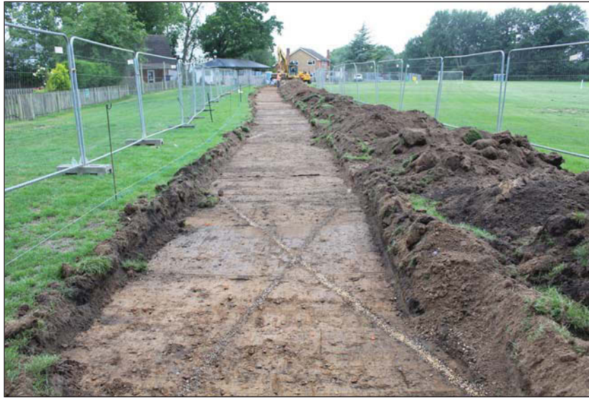
Plate 1. Haul road strip, looking E.
