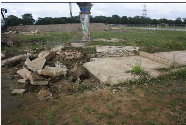
Plate 3. Demolition of building platform 1004, looking S.
