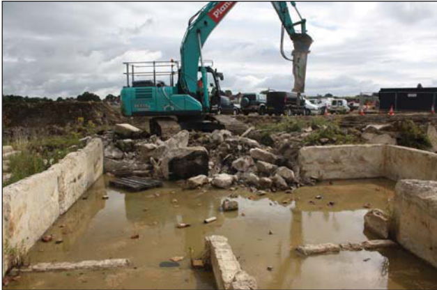
Plate 1. Demolition of command bunker 1000, looking NE.
