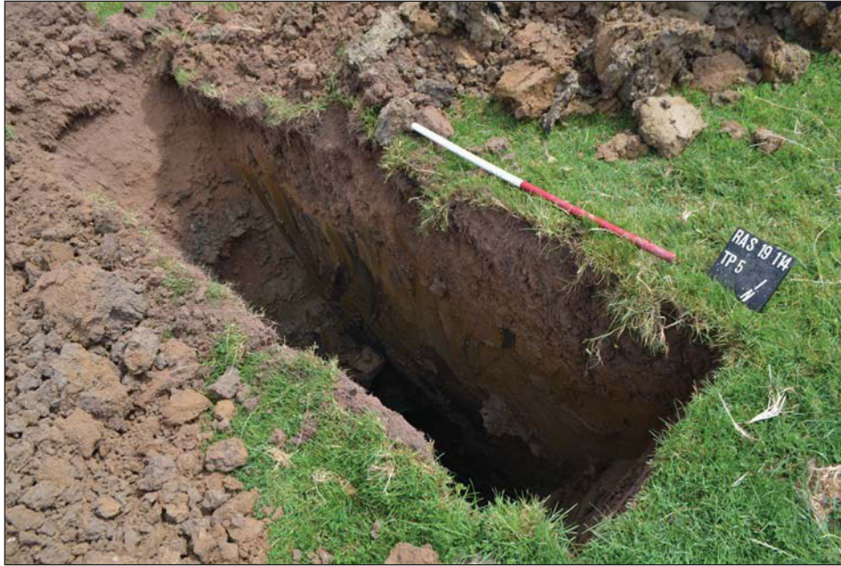
Plate 1. Geotechnical Test Pit 5
