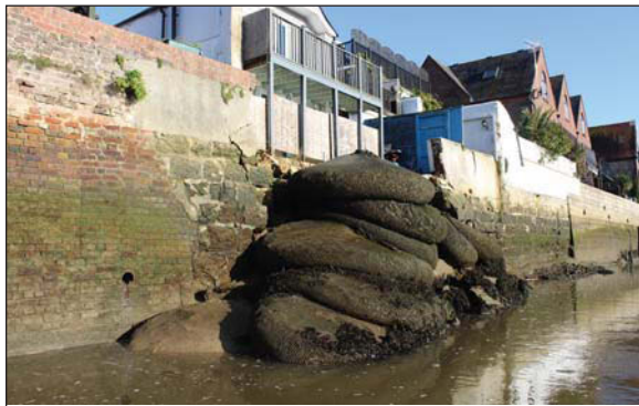
Plate 15. Wall section (c. 52-62m), looking NNE.
