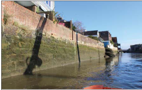
Plate 9. General view, looking NNE.
