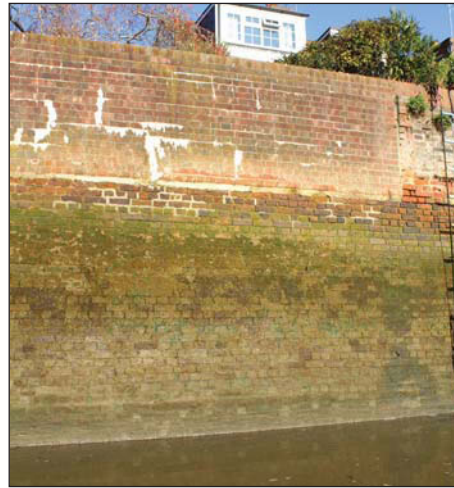
Plate 14. Wall section (c. 43m-47m), looking NNW.
