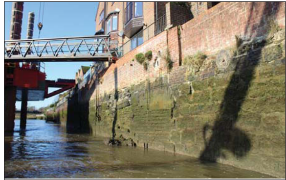
Plate 10. Wall section (c. 15m-27m), looking W.
