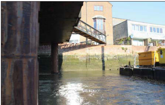
Plate 5. Wall section (c. 10m-15m), looking N.
