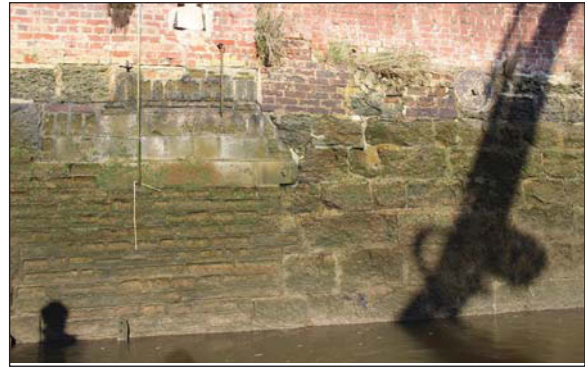
Plate 8. Wall section (c. 23m-27m), looking NNW.
