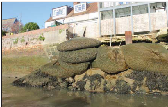
Plate 17. Wall section (c. 55m-63m), looking NW.
