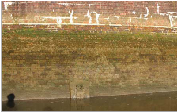
Plate 13. Wall section (c. 41m-43m), looking NNW.
