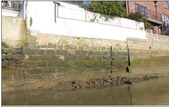
Plate 19. Wall section (c. 68m-72m), looking NNW.
