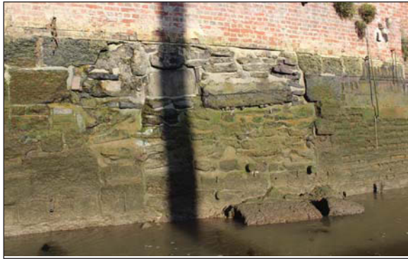
Plate 7. Wall section (c. 18m-23m), looking NNW.
