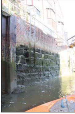
Plate 1. Wall section (c. 0-5m), looking NE.
