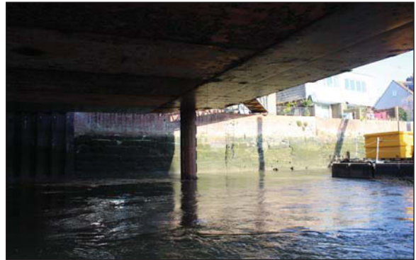
Plate 4. Wall section (c. 5m-10m), looking N.
