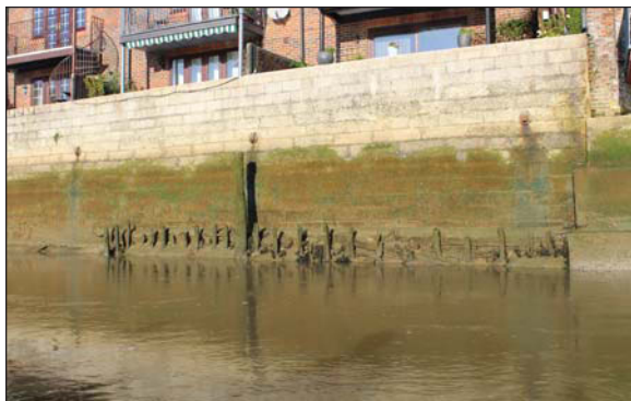
Plate 23. Wall section (c. 85m-97m), looking NNW.
