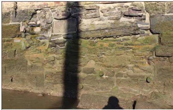
Plate 11. Wall section (c. 18m-22m), looking NNW.
