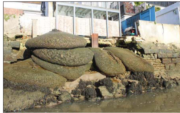
Plate 16. Wall section (c. 57m-67m), looking NNW.
