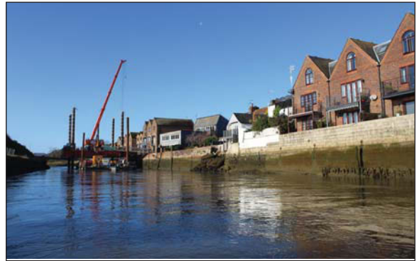
Plate 28. General view, looking E.
