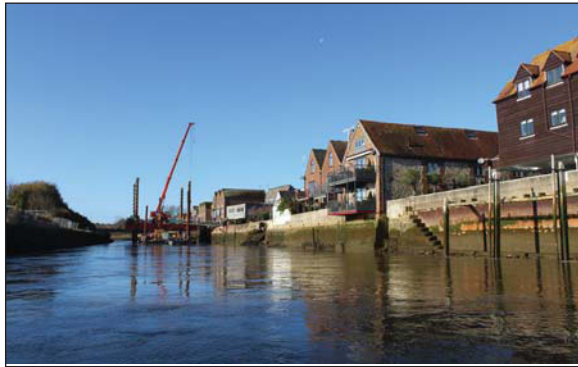
Plate 27. General view, looking E.
