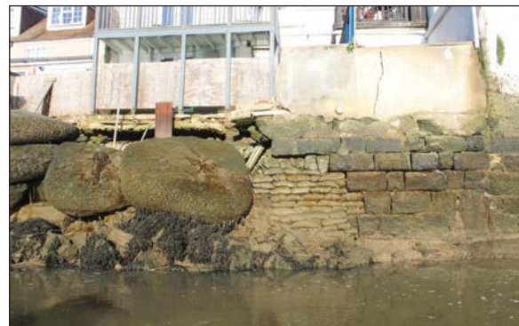
Plate 18. Wall section (c. 62m-67m), looking NNW.
