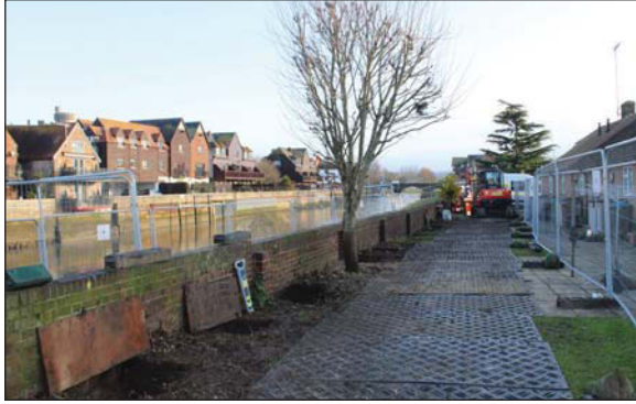
Plate 1. General view of site, looking ENE.
