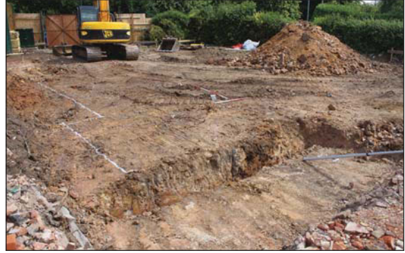
Plate 2. General view of site, looking North-east.
