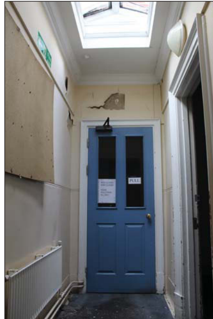
Plate 38. Corridor G-029 towards fire door for corridor G-038, looking S.
