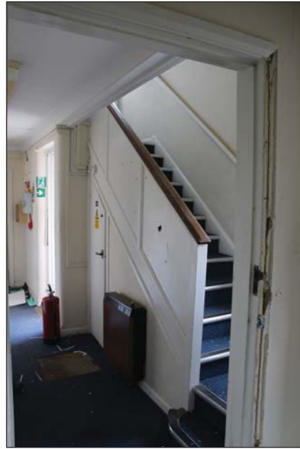
Plate 86. Lobby/Stairs G-002 towards 1st floor, looking NW.
