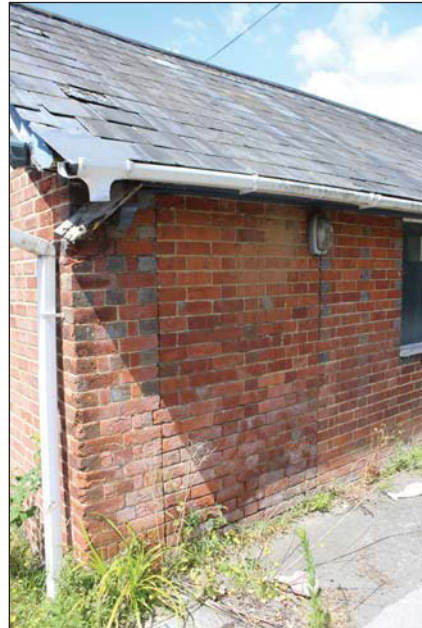
Plate 110. Towards blocked door on western front corner of Block 15, facing NE.
