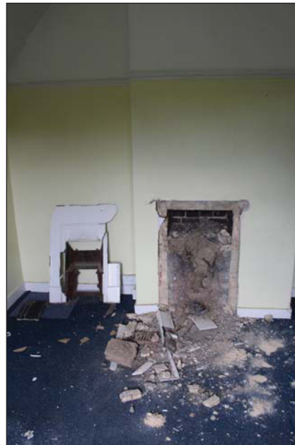
Plate 78. Office 1-003 from eastern window towards chimney, facing W.
