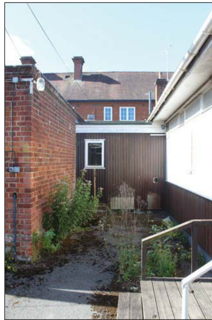
Plate 96. Alongside Block 07 and 10 towards rear of Block 01, facing S.
