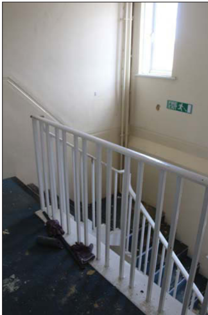
Plate 51. Lobby 1-011 towards stair well to ground floor, looking NW.
