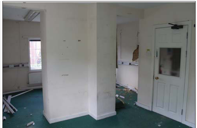
Plate 56. Office 1-020 from rear eastern corner, looking SW.
