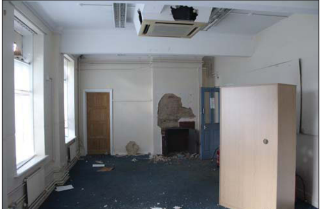
Plate 30. Office G-053, looking W.
