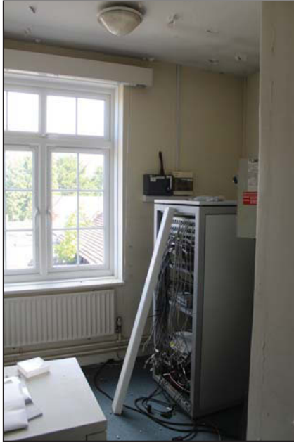
Plate 53. Entrance to office 1-015 from corridor 1-017, looking N.
