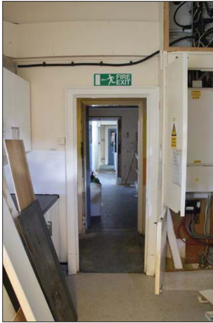
Plate 25. Kitchen from window, looking W.
