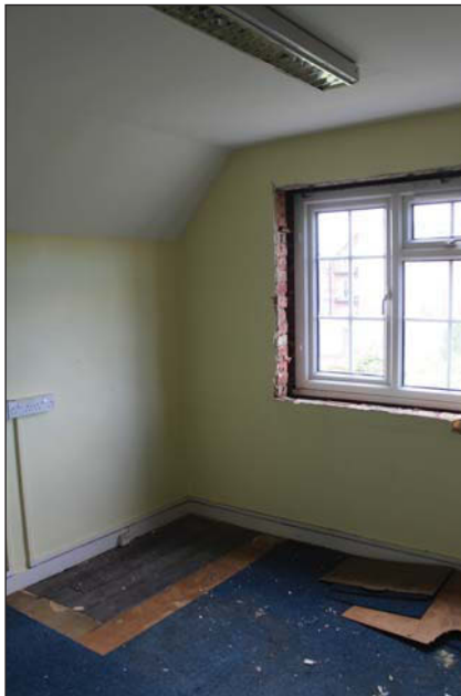
Plate 77. Office 1-006 from doorway, facing SW.
