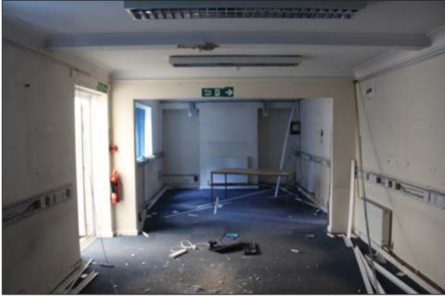
Plate 85. Office G-001, looking W.
