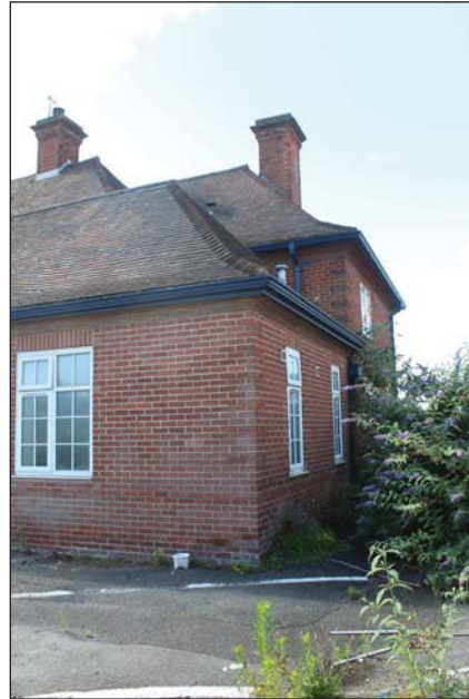
Plate 6. Rear west corner of Block 01 looking S
