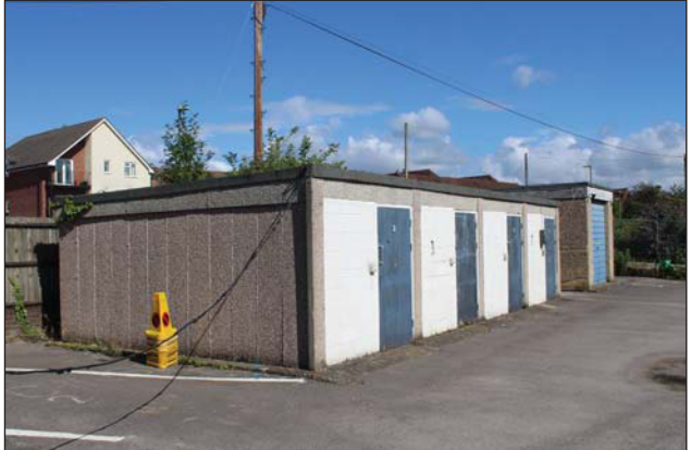
Plate 90. Block 04, facing NW.
