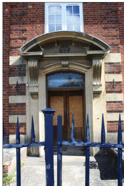
Plate 8. Front door of Block 01, looking N
