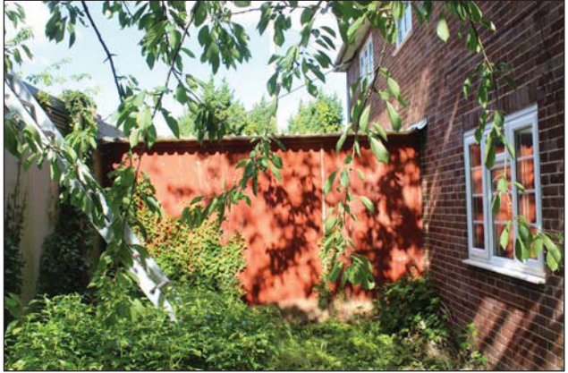
Plate 102. Rear of Block 11 and front of Block 03, facing W.
