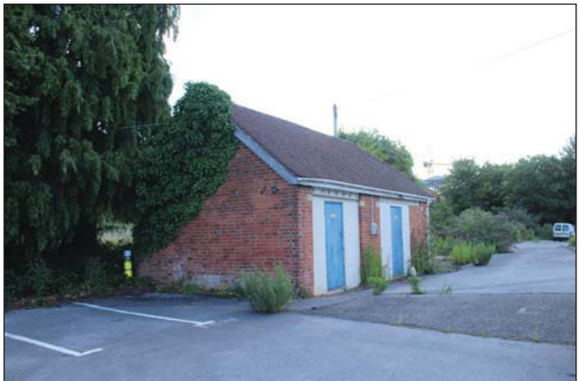
Plate 104. Front western corner of Block 12, facing NE.
