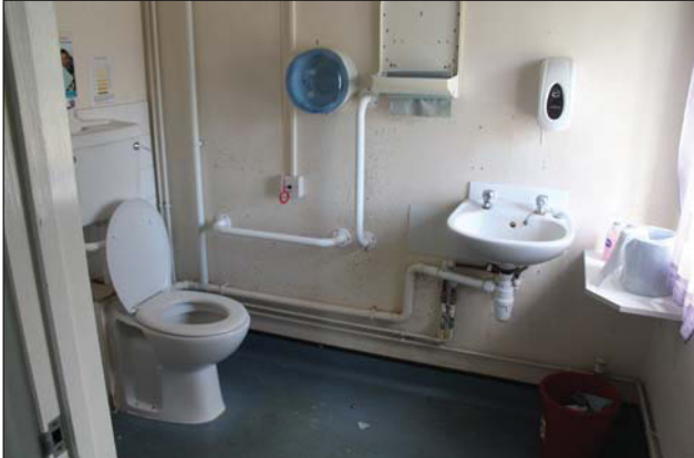
Plate 69. WC G-006, looking SW
