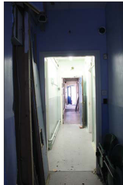
Plate 40. Store G-012 through to Lobby G-011 from eastern side entrance of Block 01, looking W.
