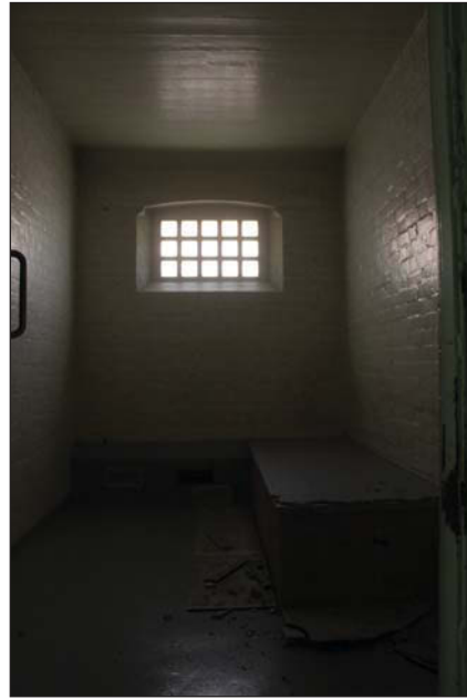
Plate 46. Entrance to cell G-021, looking W.
