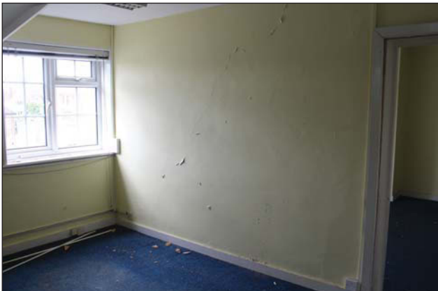
Plate 79. Office 1-004 from doorway through to office 1-005, facing SW.
