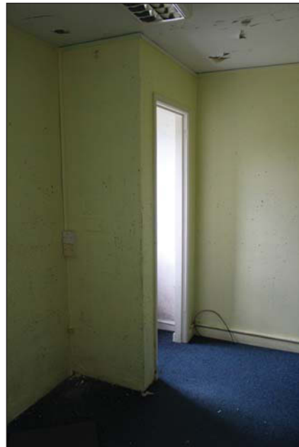
Plate 70. Office G-008 facing door, looking NE.
