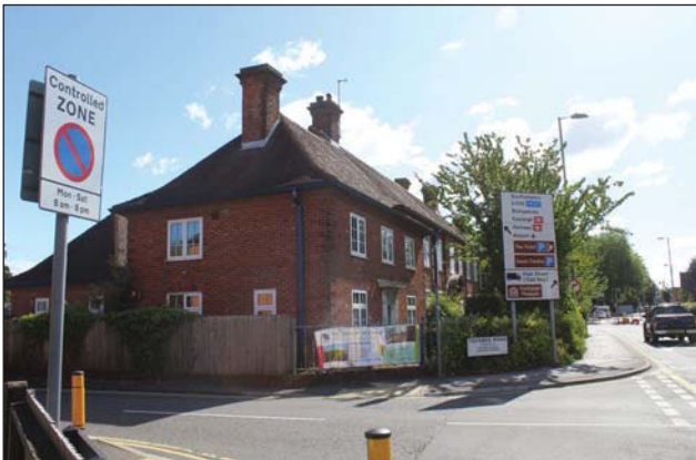
Plate 3. Front west corner of Block 01, looking NE,
