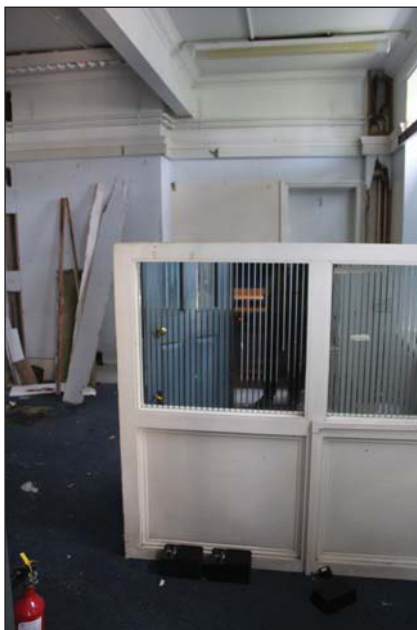
Plate 23. Office G-032 from door linking G-033, looking E.
