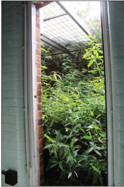
Plate 49. Entrance to exercise yard G-016 from corridor G-023, looking NE.
