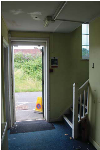
Plate 67. Looking towards western side entrance of Block 02, looking W.
