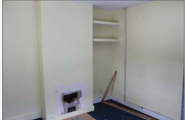
Plate 66. Office G-001 from front south eastern corner, looking NW.
