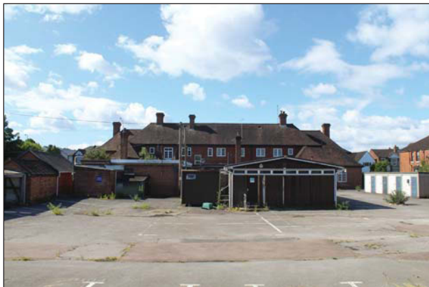
Plate 7. Rear of blocks 01, 07 and 10, looking S
