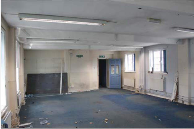
Plate 57. Office 1-008 from front south eastern corner, looking NW
