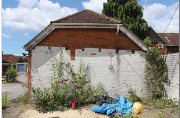
Plate 106. Towards blocked window of Block 12, facing W.
