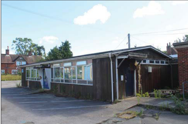
Plate 97. Front western corner of Block 07, facing NE.
