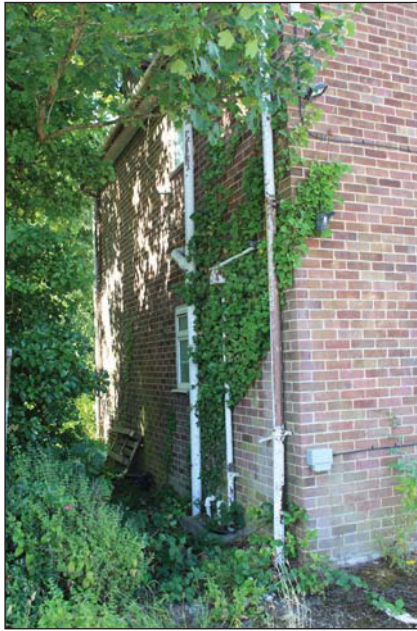
Plate 81. Along eastern side of Block 03, looking SW.
