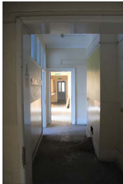
Plate 32. Corridor 5-052 looking toward lobby G-054, looking E.
