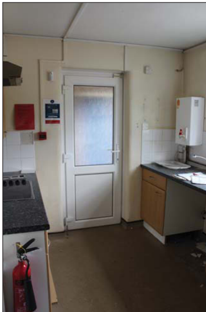
Plate 83. Kitchen G-006, looking W.
