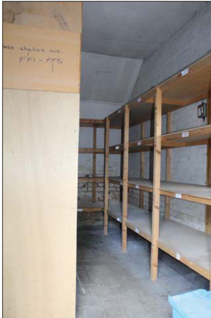
Plate 113. Store G-002 from doorway, facing NNE.
