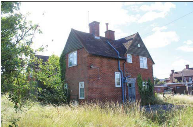
Plate 63. Rear west of block 02, 08, 13, looking SE.
