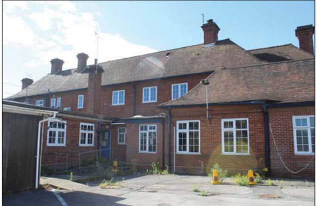
Plate 14. Rear of Block 01, looking SE.
