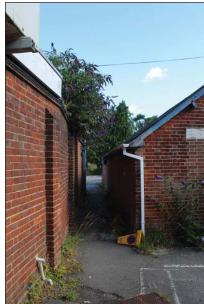
Plate 16. Alleyway between rear of Block 01 and front of Block 15 looking N.
