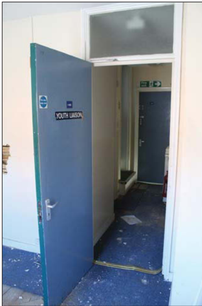
Plate 59. Doorway to office 1-002 looking through to corridor 1-005, looking ENE.
