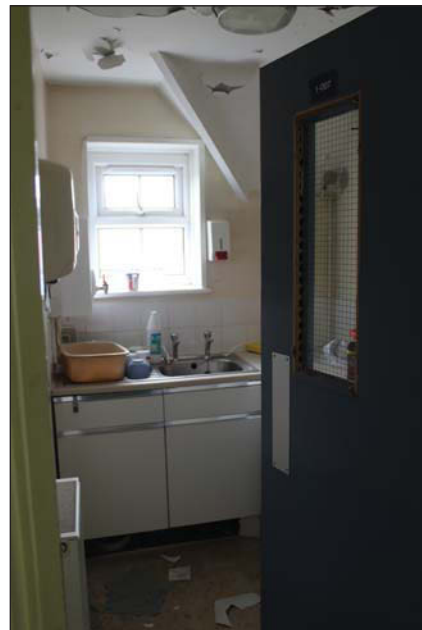
Plate 76. Kitchen 1-007 from doorway, facing NW.
