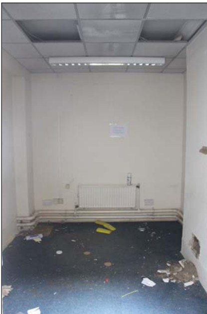
Plate 39, Office G-030 from corridor G-029, looking W.
