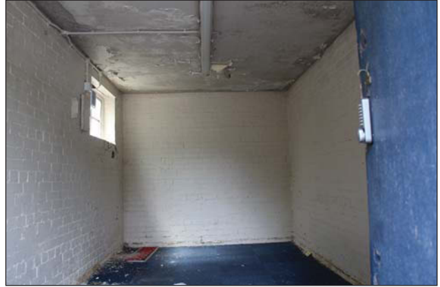
Plate 94. Lockers G-002 from doorway, facing S.
