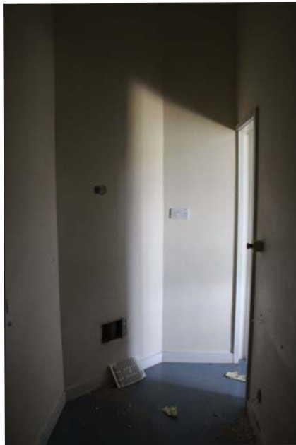
Plate 19. Office G-034A from door off lobby, looking E.
