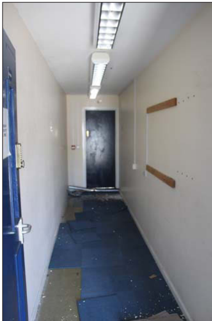
Plate 99. Store G-006A from entrance to Lobby G-006, facing S.
