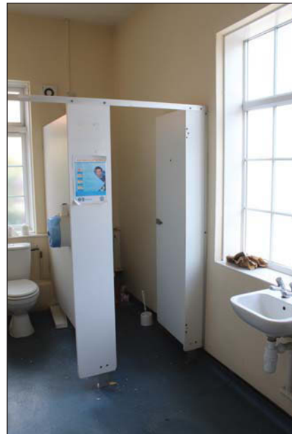
Plate 36. Ground floor WC from eastern corner of room, looking WSW.
