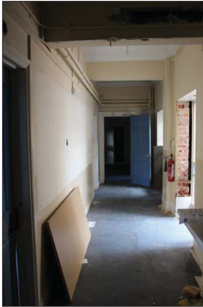
Plate 21. Lobby towards corridor G-052, looking W.
