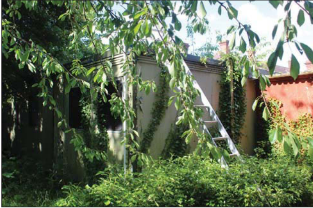
Plate 101. Rear of Block 11, facing SW.
