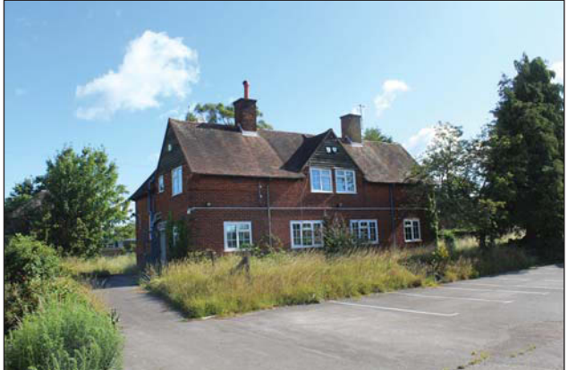
Plate 62. Front of Block 02 from east of Block 14, looking NE.
