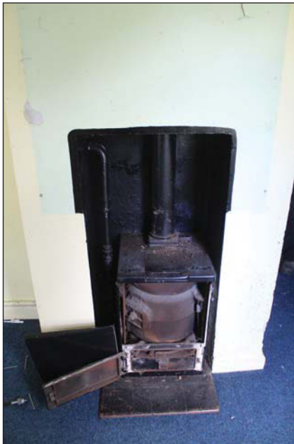
Plate 71. Fireplace in office G-008, looking S
