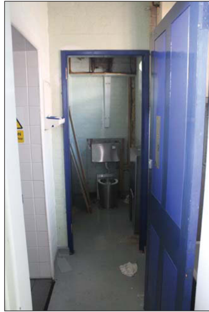
Plate 50. Entrance to WC G-015A, looking E.
