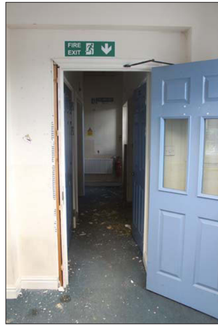
Plate 58. Doorway to office 1-008 looking through to store 1-007 and corridor 1-006, looking W.
