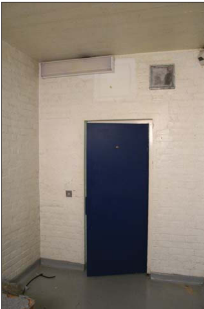
Plate 47. Doorway to cell G-021, looking NE
