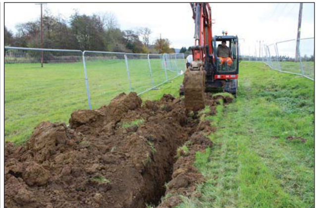
Plate 6. Ground works in North part of the project.
