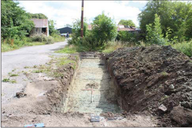
Plate 1. Trench 1, looking East, Scales: 2x1m
