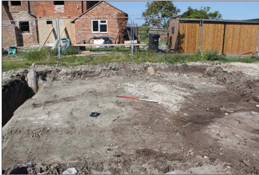
Plate 3. Stripped area over SW interior, looking WNW, Scale: 1m.
