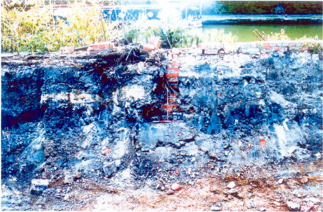
Plate 3. Removal area, wall 379 and foundation 380 of canalside workshop, looking south east, scales 0.5m.
