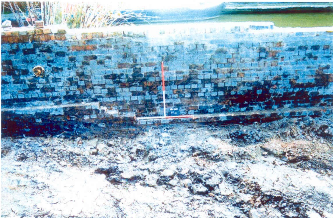
Plate 4. Removal area, canal wall 377, looking south, scales 1m.
