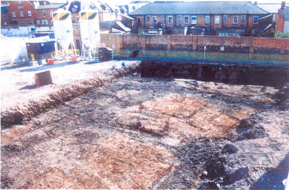
Plate 2. Borrow pit strip, looking south, scales 2m and 1m.
