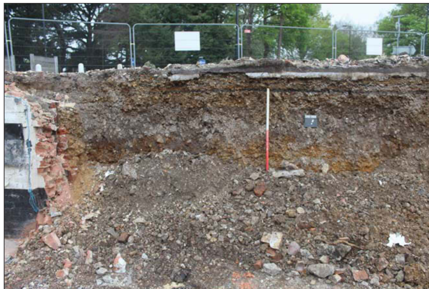
Plate 1. Exposed ground section, behind basement wall, looking North, Scale: 1m.
