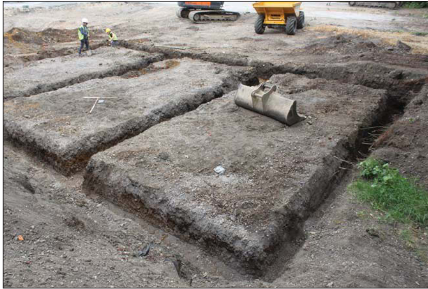
Plate 1. Foundation trenches of block 1, looking North East, Scales: 2x1m.
