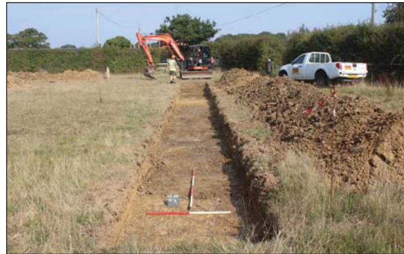
Plate 4. Trench 7, looking North-north-east. Scales: 2m, 1m and 0.30m.
