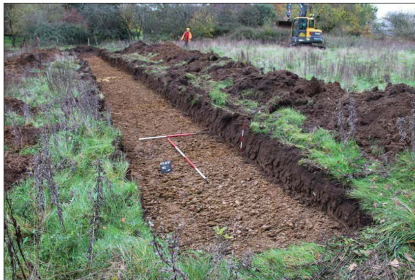
Plate 3. Trench 3, looking North West, Scales: horizontal 2m and 1m, vertical 0.3m.
