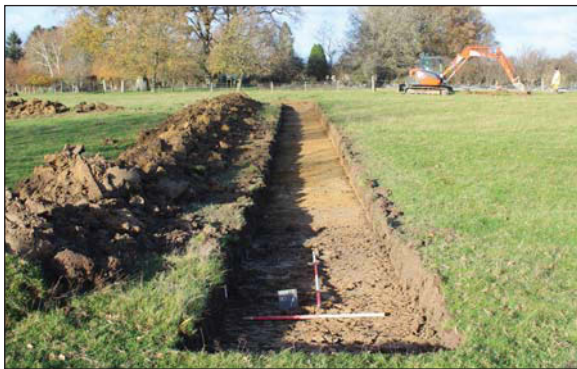
Plate 3. Trench 7, looking North-north-west. Scales: 2m, 1m and 0.3m.
