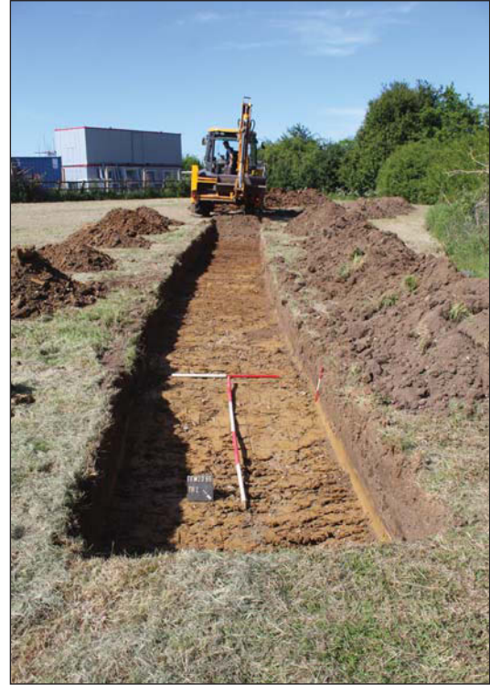
Plate 2. Trench 2, looking SW, Scales: horizontal 2m, 1m, vertical 0.3m.
