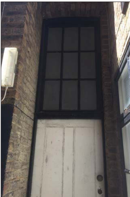
Plate 11. Window above detail, looking Southwest.
