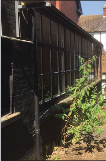
Plate 9. Oblique of long window, looking West-northwest.
