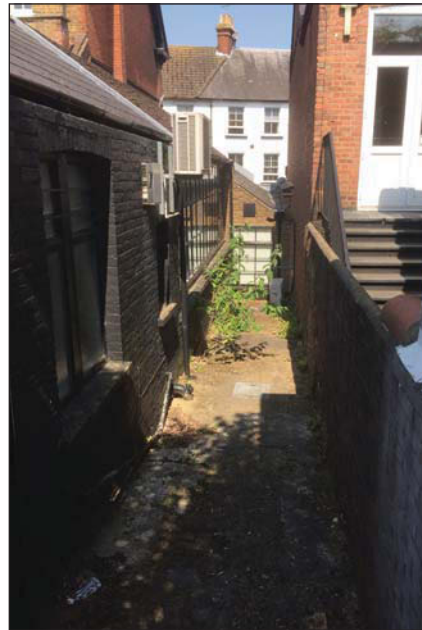
Plate 2. View down length of building, looking Northwest.
