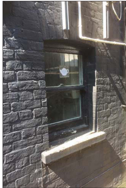
Plate 8. Window detail, looking West.
