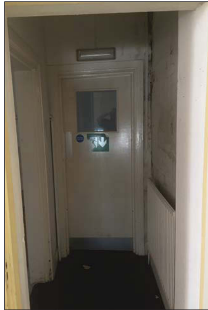
Plate 18. Corridor, looking Southeast.
