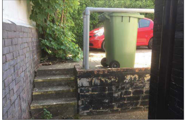
Plate 6. Step detail, looking Southeast.
