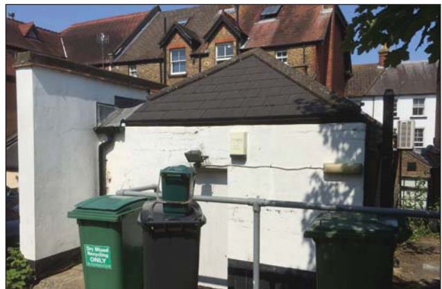
Plate 4. Rear wall showing door, looking Northwest.
