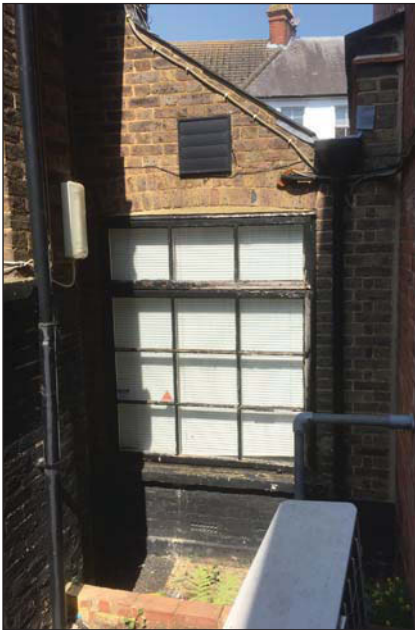
Plate 7. Window detail, looking Northwest.
