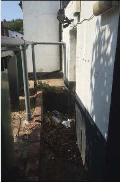
Plate 5. Along rear wall, looking Southwest.
