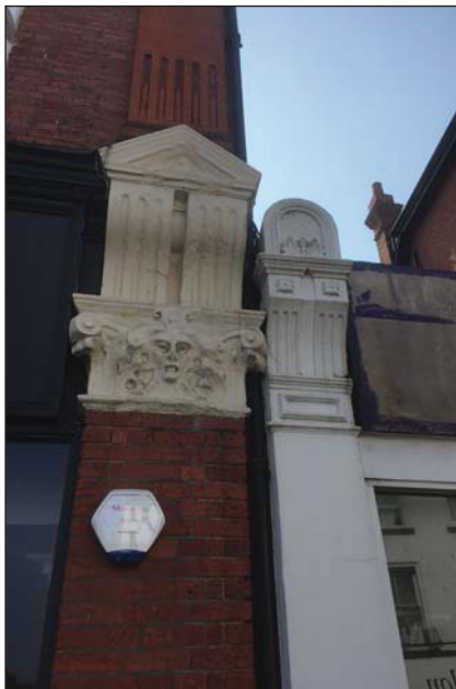
Plate 3. Pilaster detail, looking Southeast.
