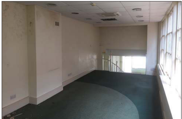
Plate 16. Room 2, view to stairs, looking West.
