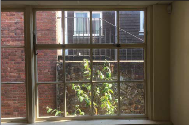
Plate 17. Room 2, window detail, looking Northeast.
