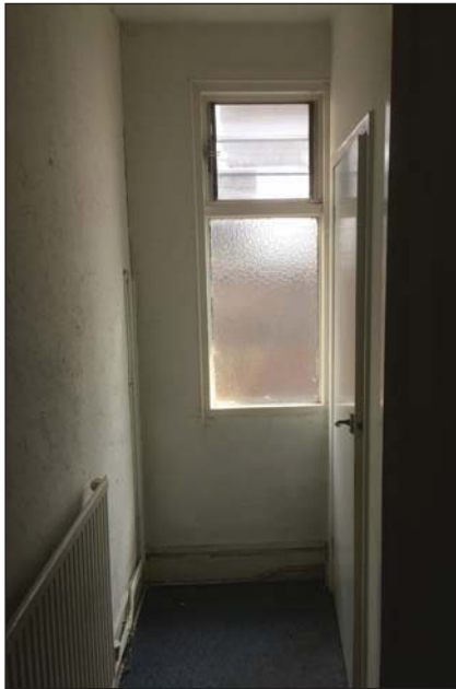
Plate 21. Room 4, window detail, looking Northeast.
