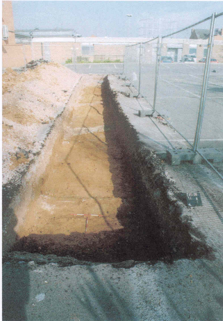
Plate 1. Trench 1, looking north, horizontal scales 0.5m.
