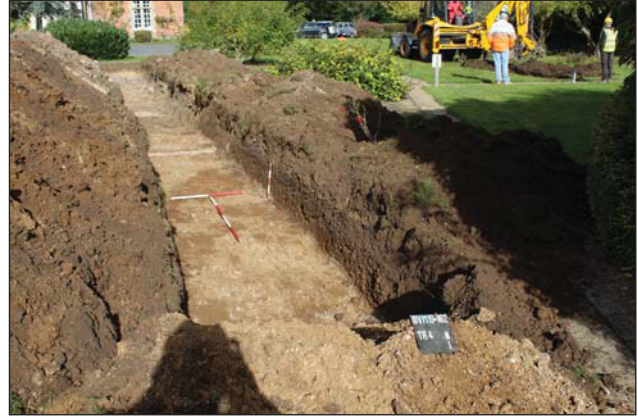
Plate 2. Trench 4, looking North east, Scales: 2m, 1m and 0.5m.
