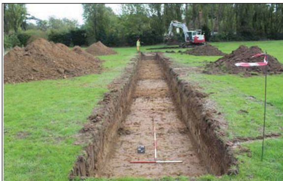
Plate 5. Trench 10, looking East-south-east. Scales: 2m, 1m and 0.50m.
