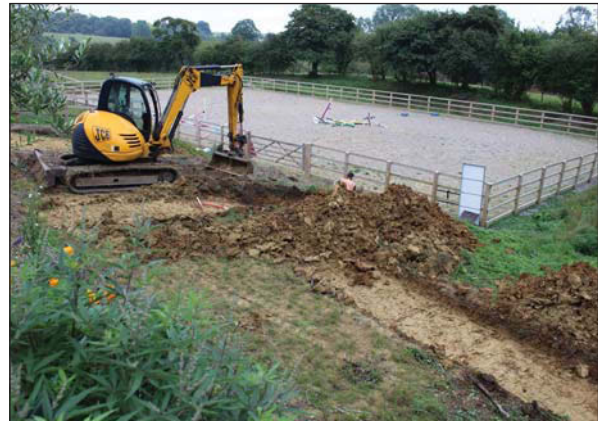
Plate 3. Trench at the top of the terrace slope, looking South East.
