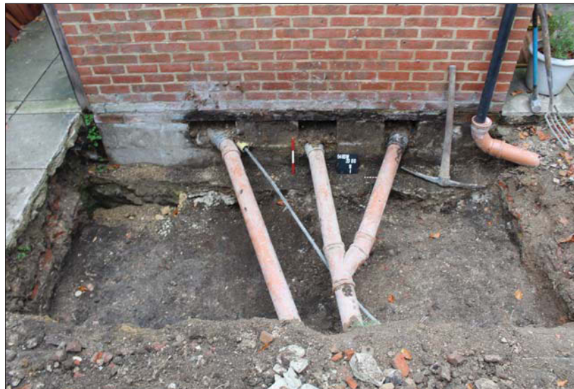
Plate 2. Finished excavation, exposing made ground (56).
