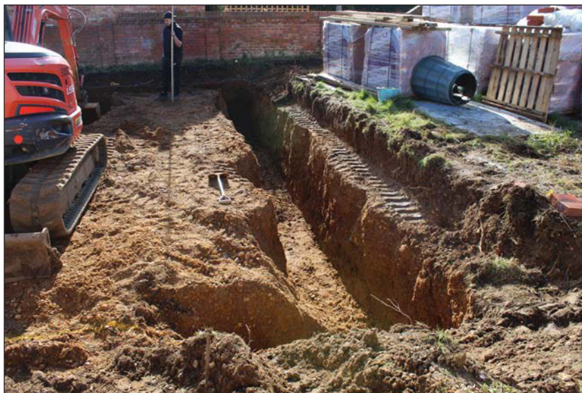
Plate 4. Excavation of footings looking South East
