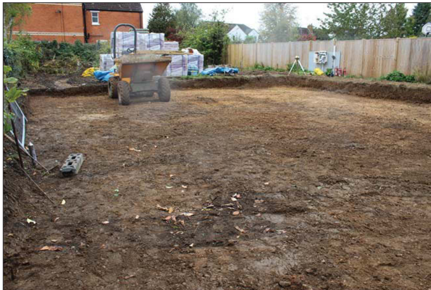
Plate 2. Completed strip for formation level, looking South East
