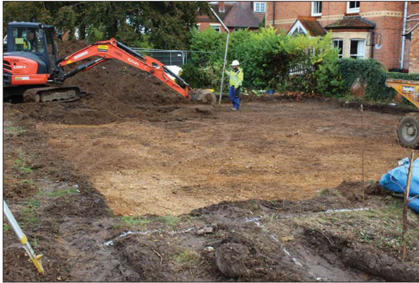
Plate 1. Stripped area to formation level in progress, looking North East
