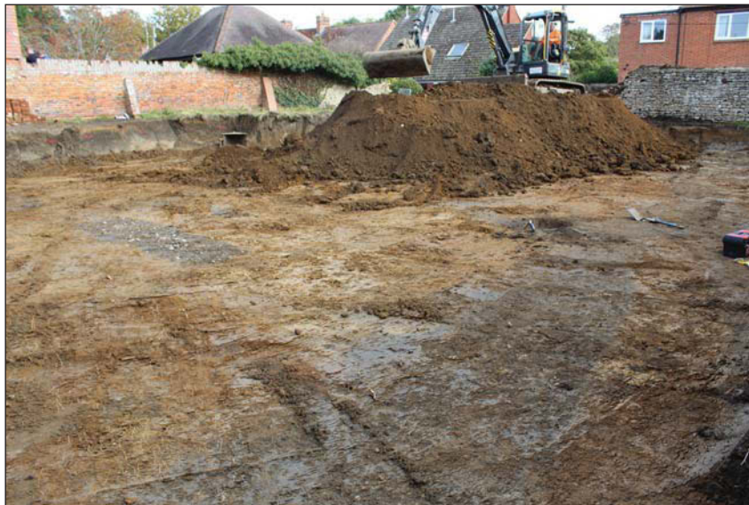
Plate 4. Formation level stripped in western and southern areas, looking North East.
