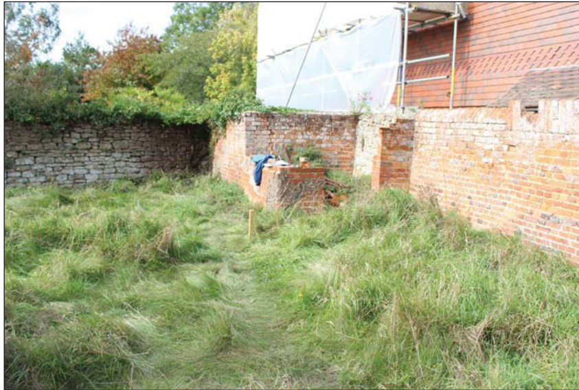
Plate 1. Remnant of structure in northwest corner of site, looking North East
