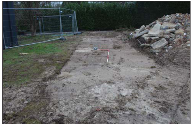
Plate 4. General site shot, access road looking North East, Scales: 2m and 1m.
