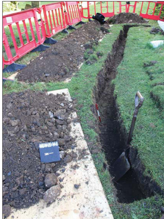
Plate 2. Route of new drainage trench, looking W; Scale: vertical 0.3m.
