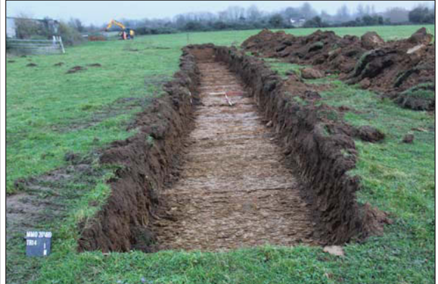
Plate 6. Trench 14, looking South, Scales: 2m and 1m.
