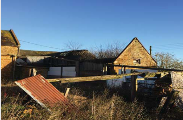
Plate 9. Building D, Looking North East.
