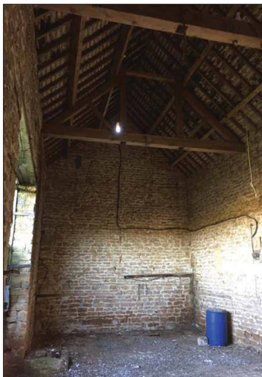
Plate 20. Building C, Looking East.
