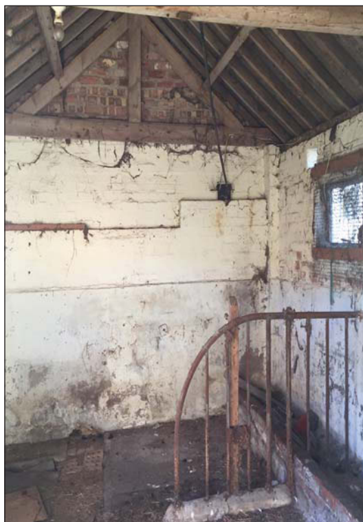
Plate 14. Room A2, Looking South.
