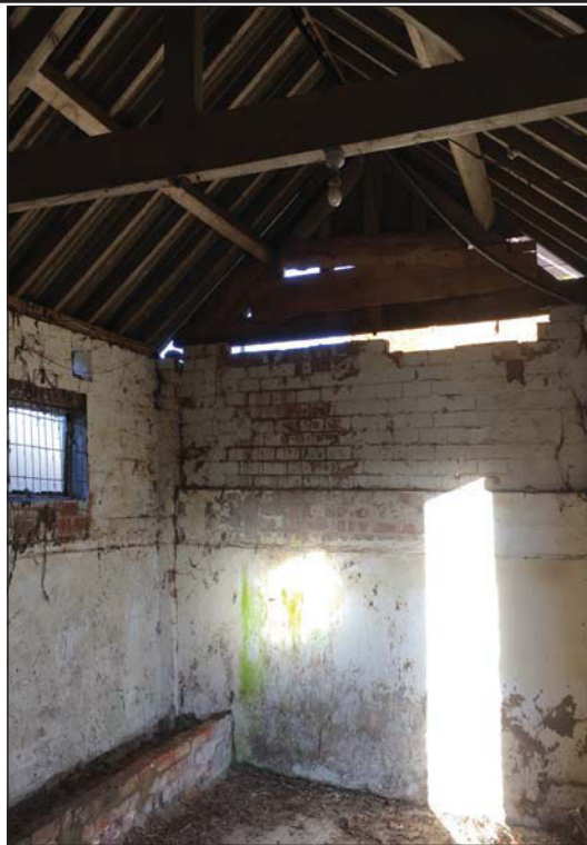
Plate 15. Room A2, Looking North North West.
