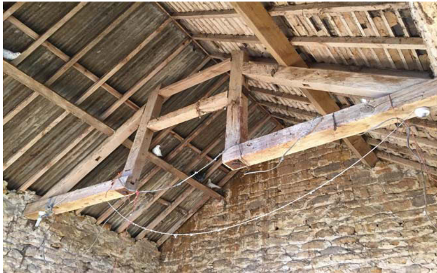
Plate 17. Building B Showing Roof Structure, Looking North West.
