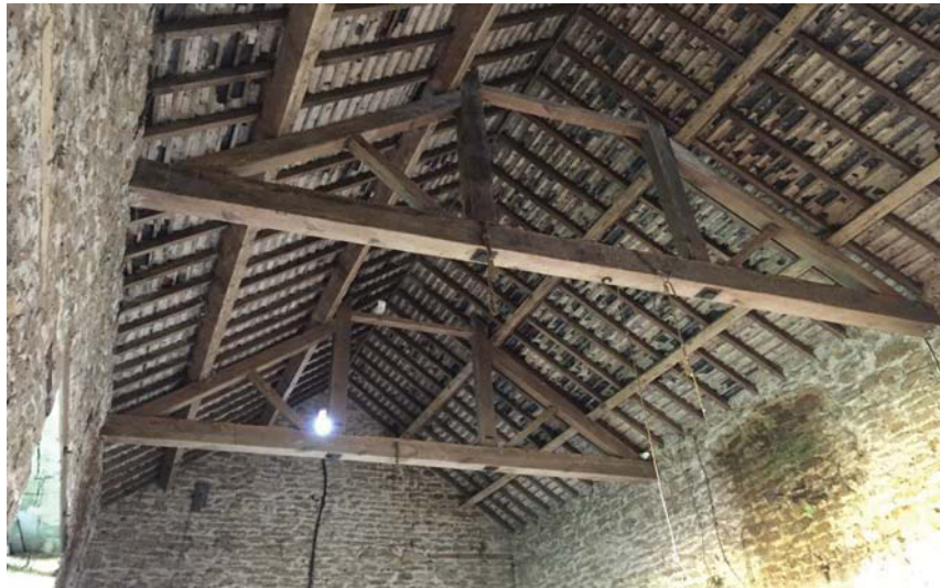
Plate 21. Building C Showing Roof Structure, Looking East South East.
