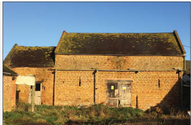
Plate 8. Buildings B and C, Looking North.
