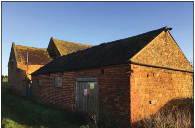
Plate 4. Building A, Looking North North East.
