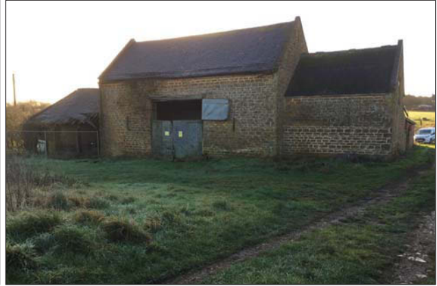
Plate 6. General view of site, Looking South South East.
