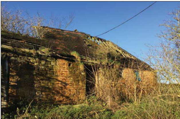
Plate 11. Building D, Looking North North West.
