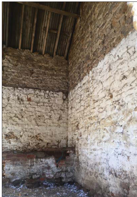
Plate 16. Building B, Looking North.
