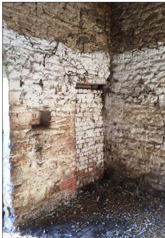
Plate 18. Building B Showing Blocked Doorway, Looking South West.
