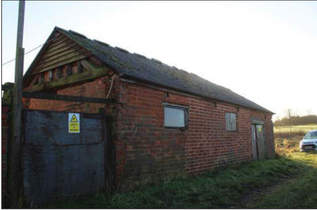
Plate 5. Building A, Looking South East.
