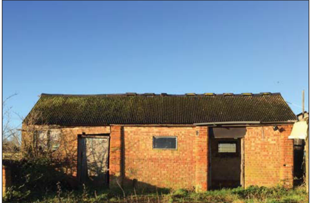
Plate 10. Building A, Looking West.
